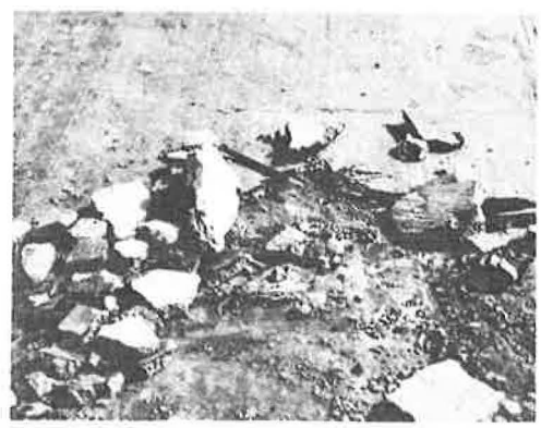
Figure 11. Soil-cement base with top 3/4 in. broken away, Iowa 37.
