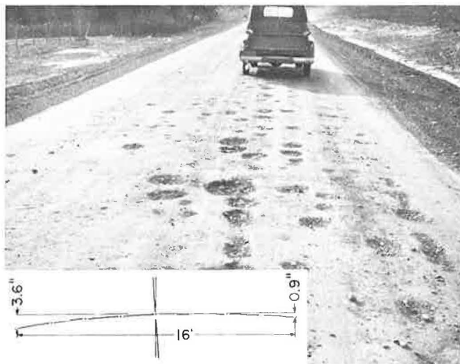
Figure 9. Potholing on uphill side of soil-aggregate road.
