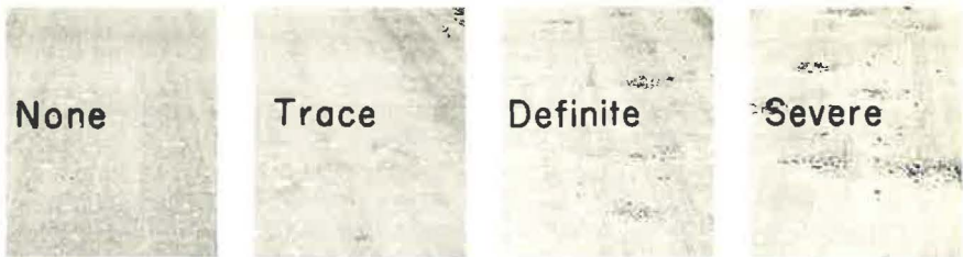
Figure 2. Visual definition of pothole severity.
