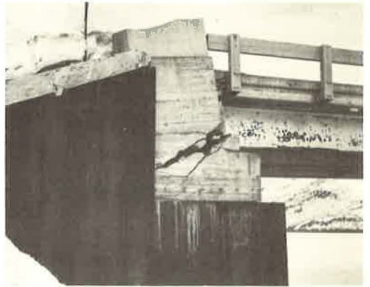
Figure 6. Abutment of Valdez Glacier Stream bridge.
