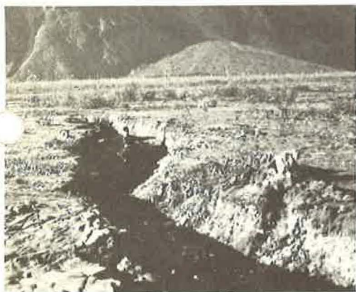
Figure 12. Crack near Mile 63, Copper River Highway, approximately 10 ft wide, 5 ft deep and 300 ft long; note fine sand ejected during quake.
