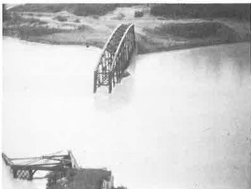
Figure 17. Steel truss bridge at Mile 28, Copper River Highway, with center pier missing; span tipped over as a result of movement of river ice.
