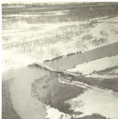
Figure 11. Aerial view of 37.2 Mile bridge, Copper River Highway, showing evidence of vertical movement on right-hand abutment, and ground cracks on right.
