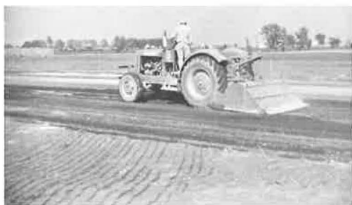
Figure 13. Mixing soil-lime with rotary mixer.
