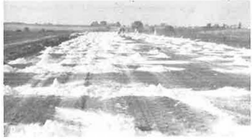
Figure 8. Opening bags of lime.
