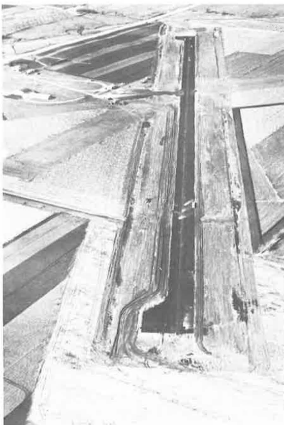
Figure 15. Airstrip with subbase, MC-0 cure, and asphaltic concrete base.
