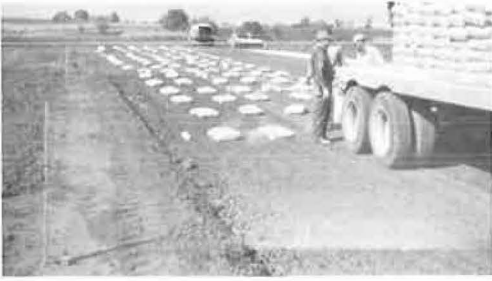
Figure 7. Unloading and spotting bagged lime.
