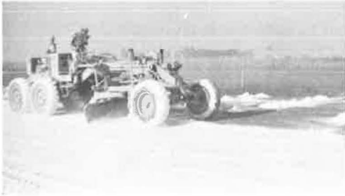
Figure 9. Spreading bagged lime with motor grader.
