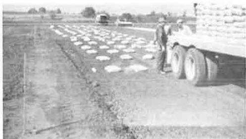
Figure 7. Unloading and spotting bagged lime.
