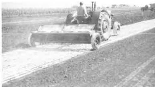
Figure 10. Spreading lime with drill spreader.
