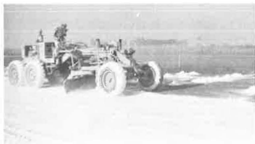
Figure 9. Spreading bagged lime with motor grader.
