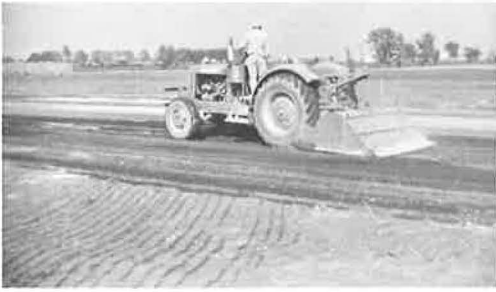
Figure 13. Mixing soil-lime with rotary mixer.
