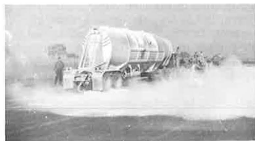
Figure 11. Spreading bulk lime with a long sweep discharge elbow attached to bulk transport; only a slight amount of dusting and air-borne lime.
