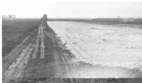
Figure 12. Completed spread from one load of bulk lime directly down runway edge (note uniformity of spread).
