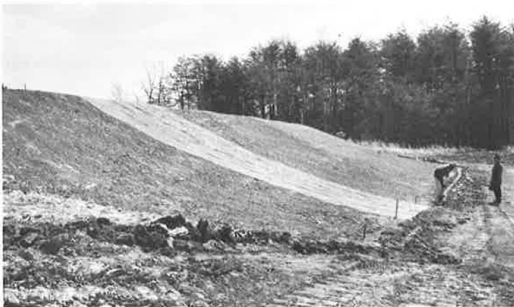
Figure 1. Laying jute and mulchnet on embankment.
