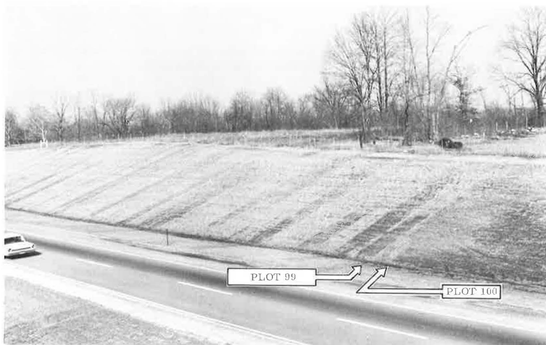
Figure 4. East side of cut section, March 1962.
