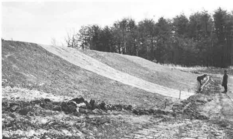
Figure 1. Laying jute and mulchnet on embankment.
