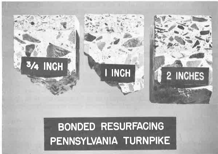
Figure 6. Pavement sections cut from Pennsylvania Turnpike.
