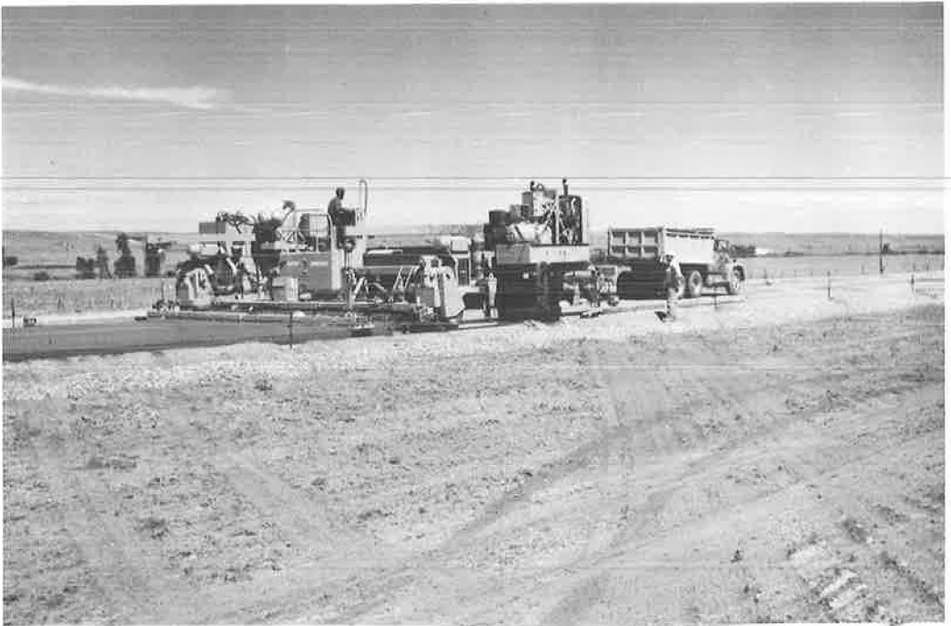
Figure 5. Guntert-Zimmerman slip-form paver.
