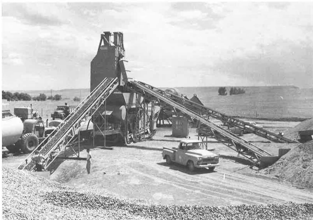
Figure 3. Concrete batching and mixing plant.
