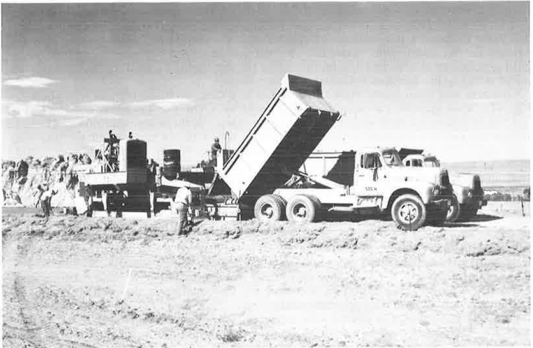
Figure 4. Dump trucks for hauling mixed concrete.
