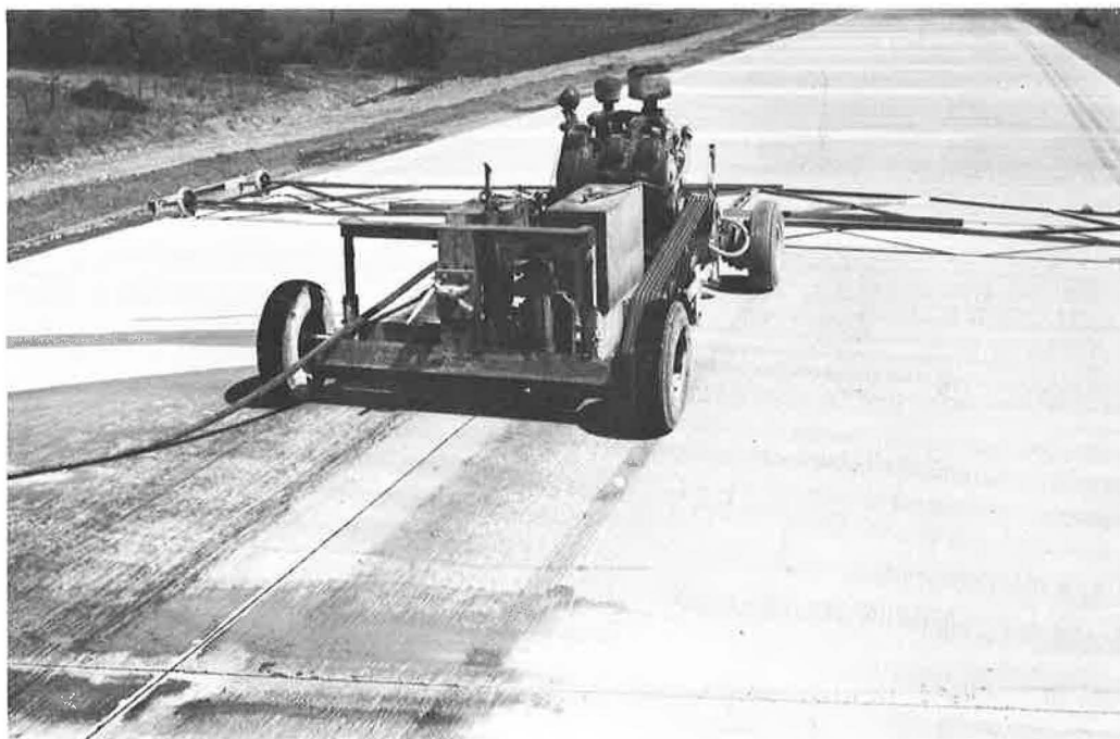
Figure 7. Equipment for sawing longitudinal joint.
