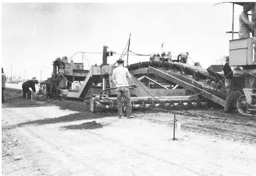
Figure 14. Prototype of combined-unit slip-form paver.
