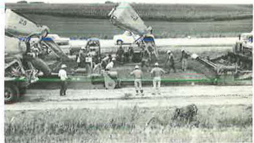
Figure 7. Device developed for paving I-80 project in Iowa.
