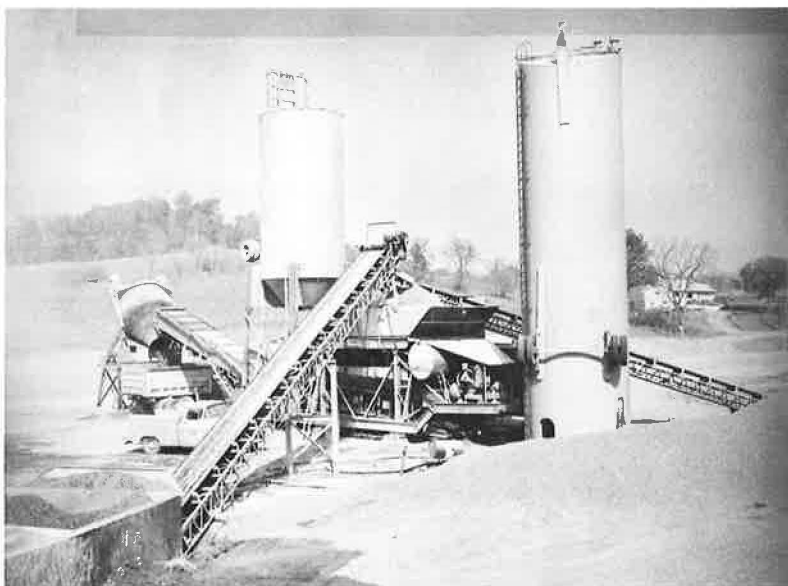
Figure 3. Central mix plant.
