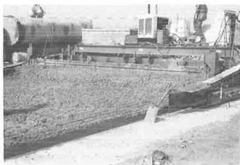
Figure 6. Second Rex slip-form paver.
