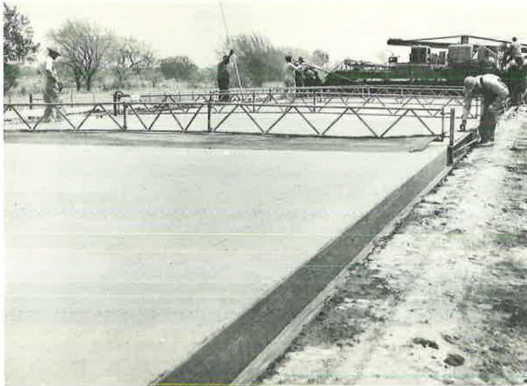
Figure 5. Finished slab on twin slip-form project, I-40.
