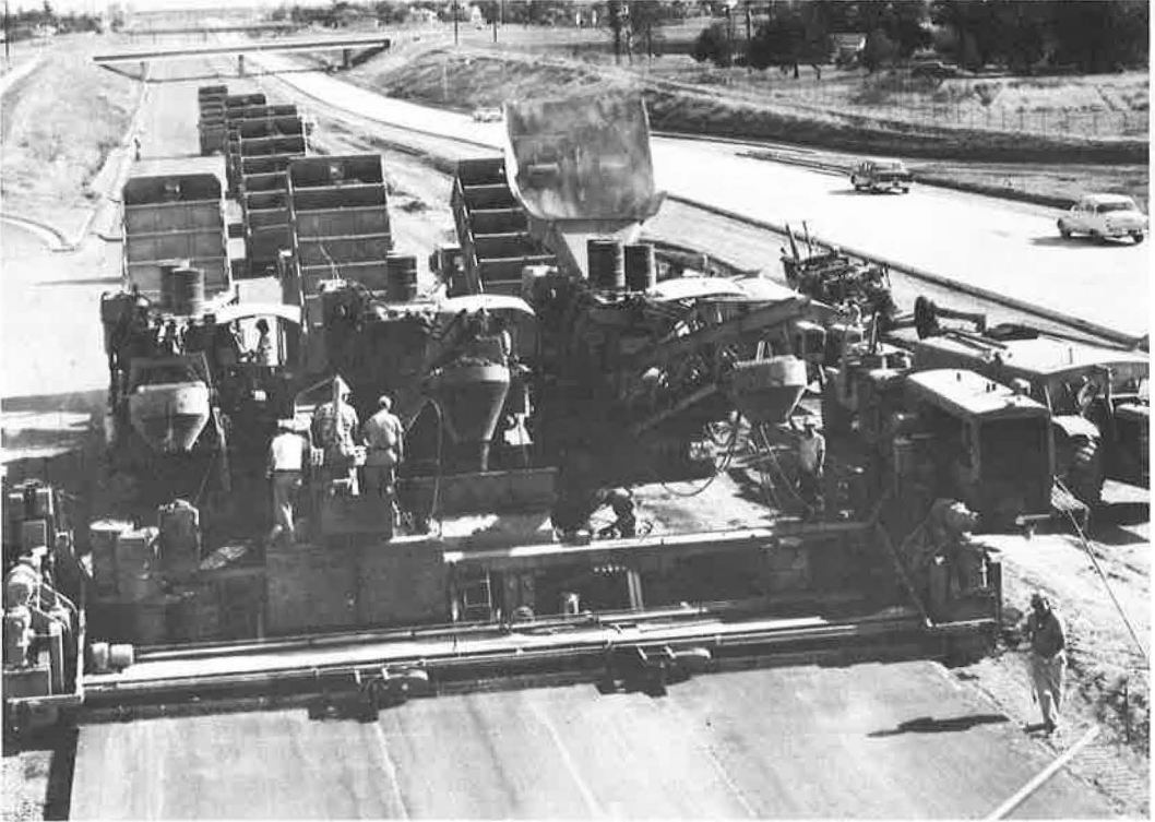
Figure 6. Thirty-six-foot highway slip-form paver.
