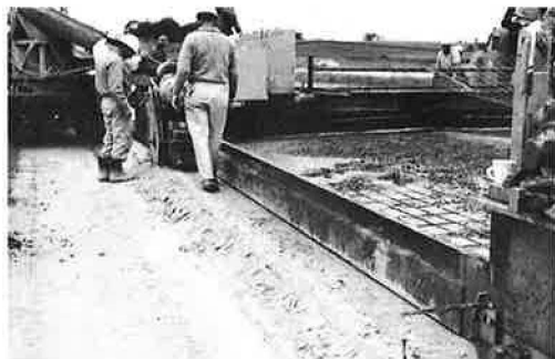
Figure 8. Special 45-ft length of form to guide crawler-mounted screw spreader.
