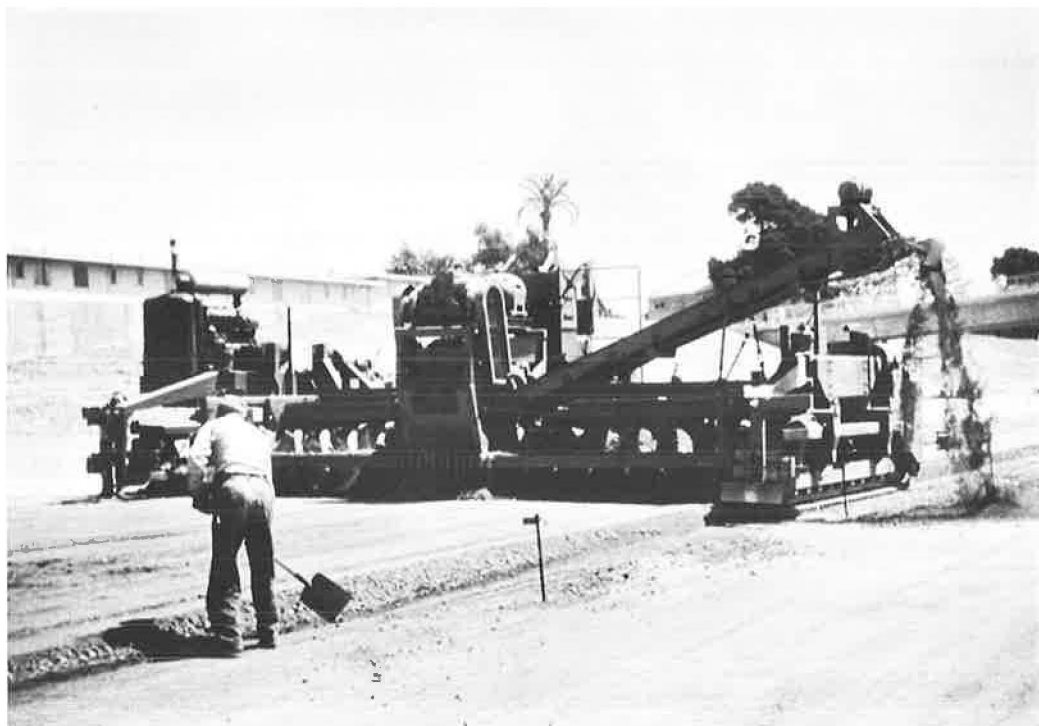
Figure 8. Full-width (28-ft) self-propelled subgrader on crawlers, controlled from reference wire.
