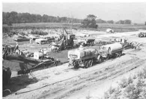
Figure 4. Rex slip-form paving train.
