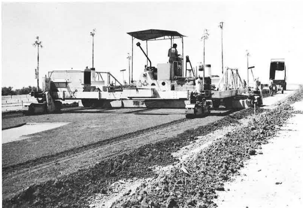
Figure 10. Accurately controlled thickness of loose material placed 28 ft wide by machine.
