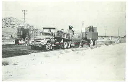
Figure 12. Central-mixed concrete hauled in dump trucks feeding 36-ft Guntert-Zimmerman slip-form paver.
