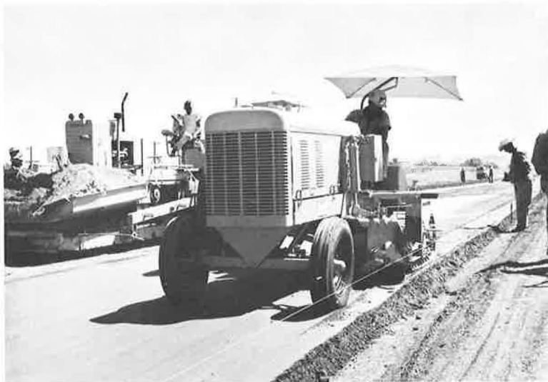
Figure 2. Electronically controlled form-grader cutting trench at edge of subbase.
