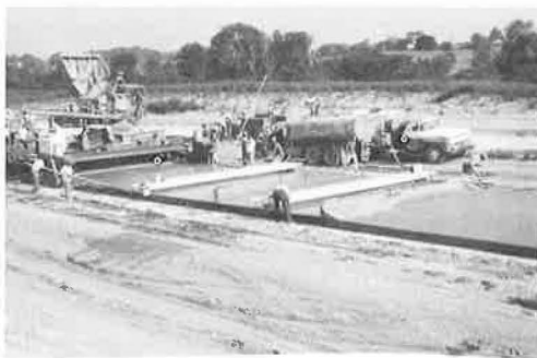
Figure 8. Finishing operations behind second paver.
