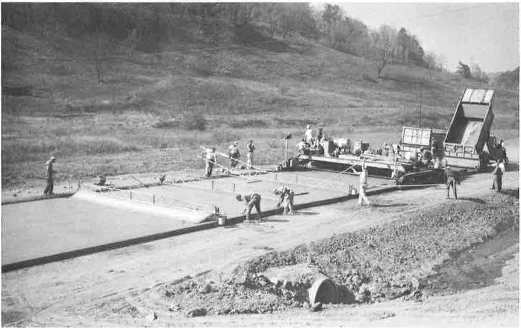
Figure 6. Finishers correcting surface and edging concrete along forms.
