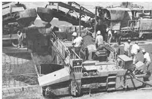
Figure 17. Blaw-Knox slip-form paver operating on ditch invert in southern California.
