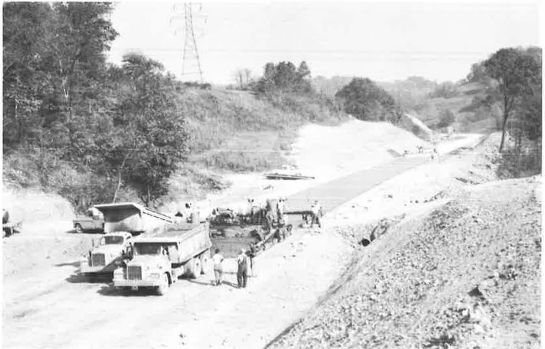
Figure 8. Application of membrane curing material.
