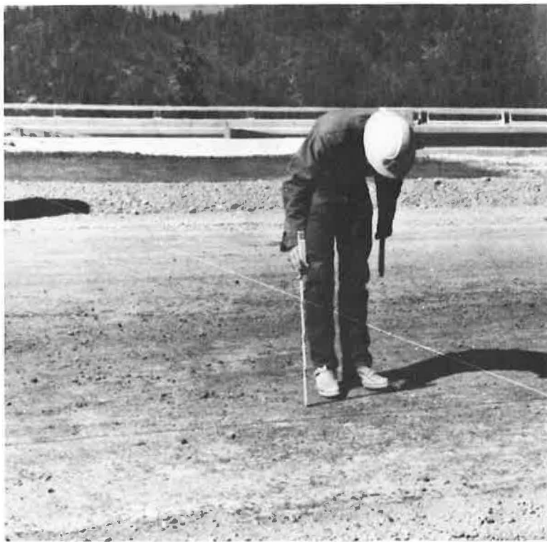
Figure 10. Subgrade measurement from taut string line.
