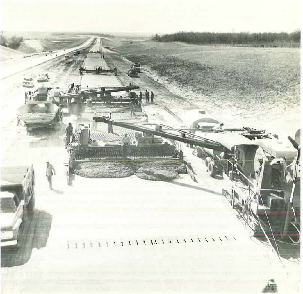
Figure 1. Two Rex slip-form pavers in use on I-40 in Oklahoma.
