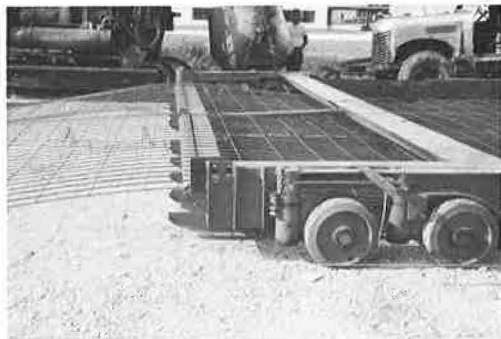
Figure 3. Sled attachment on Rex slip-form paver used in unsuccessful single-lift process.
