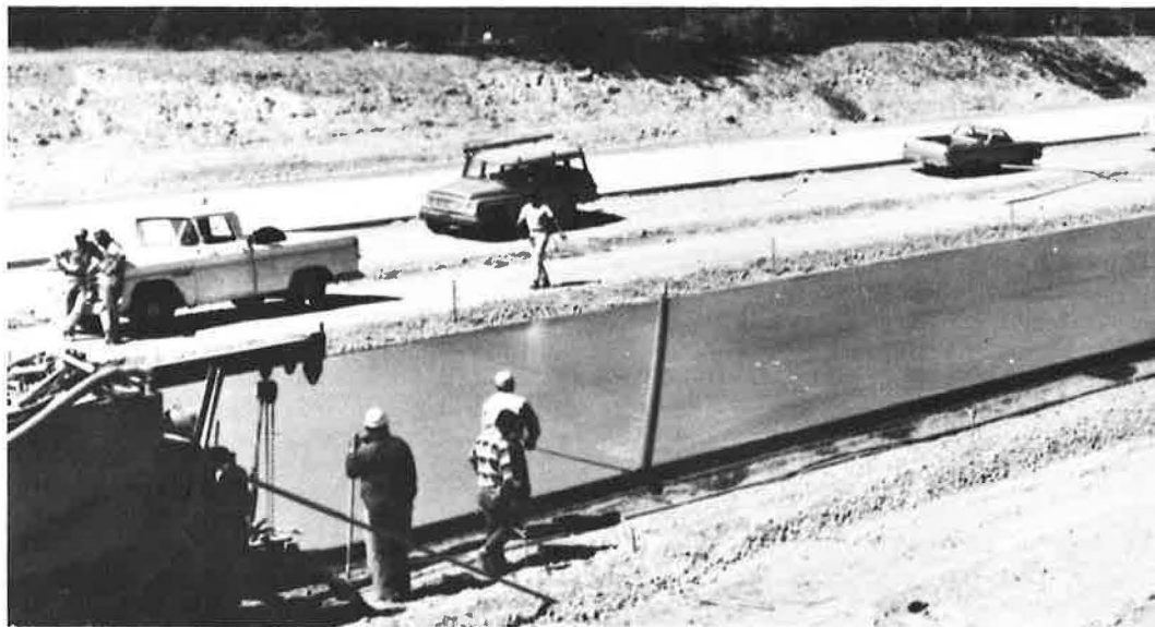
Figure 15. Pipe float procedure.
