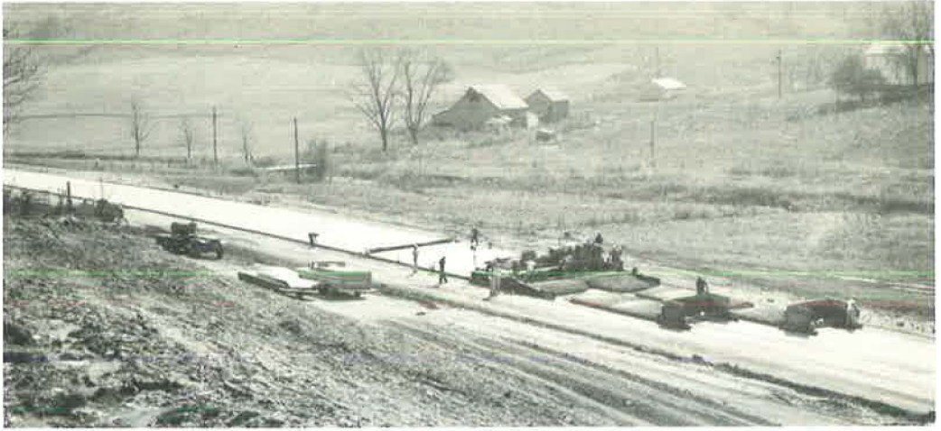
Figure 4. Uniform spread of concrete ahead of slip-form paver.
