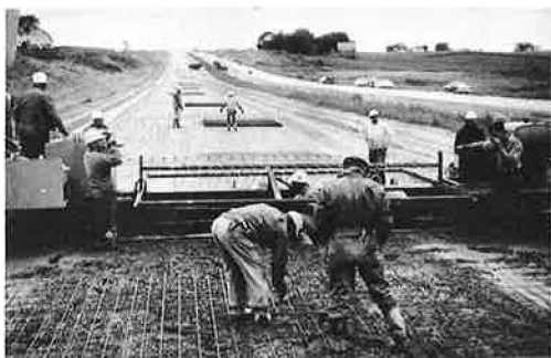
Figure 9. Placing mesh on first lift of concrete.
