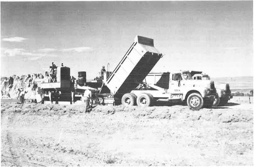
Figure 4. Dump trucks for hauling mixed concrete.
