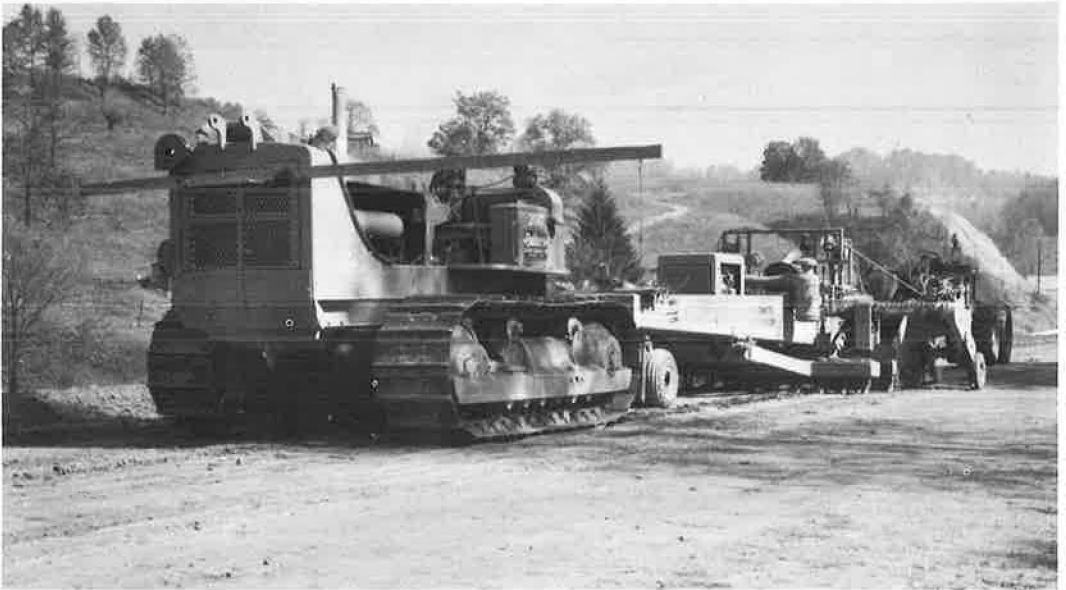
Figure 2. Subgrade approximately 1 in. above grade.
