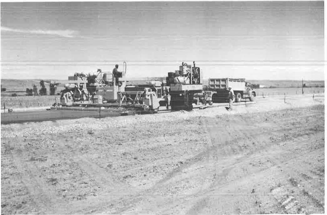
Figure 5. Guntert-Zimmerman slip-form paver.
