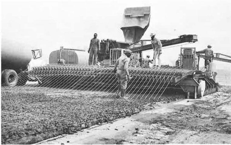
Figure 3. Mesh carried by front paver.
