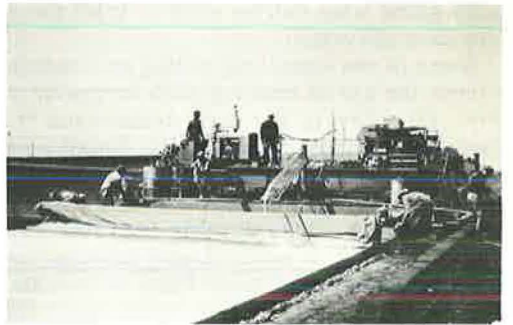
Figure 14. Koehring-Johnson experimental slip-form operating in Oklahoma in 1963.
