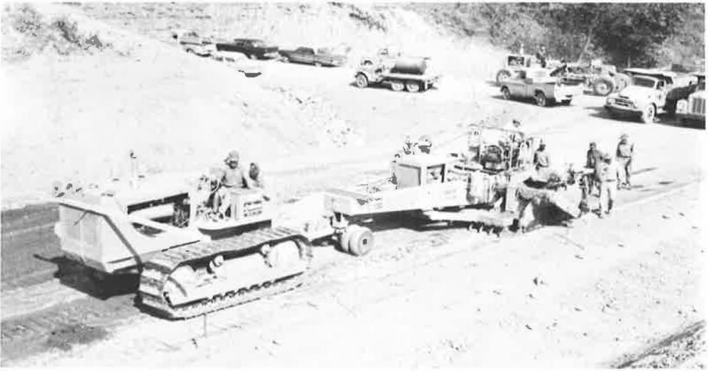
Figure 1. Gurries automatic roadbuilder.
