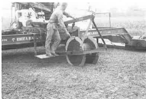
Figure 5. Tie bar placer of lead paver.
