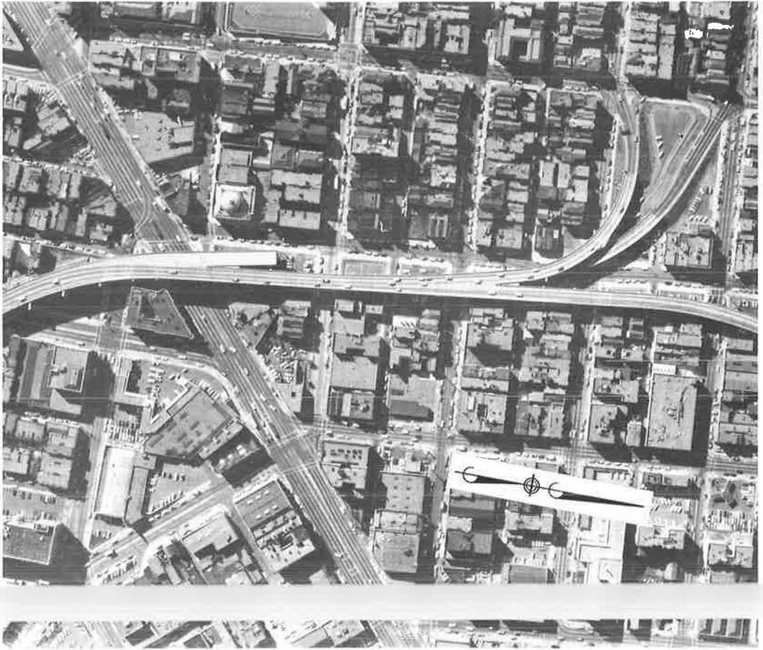
Figure 5. Central Skyway, San Francisco.
