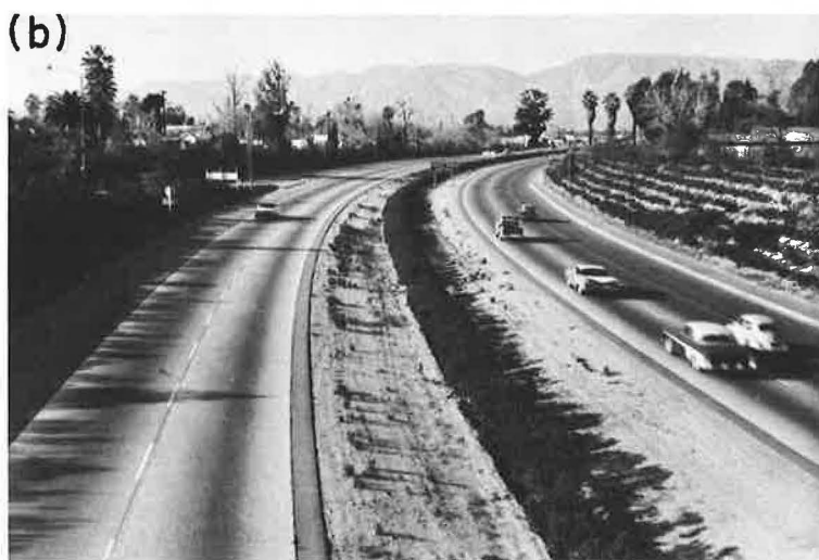
Figure 23. Section 31: (a) near south city limits of Colton (accident rate, 1.07); and (b) near Colton Ave. (accident rate, 1.62).
