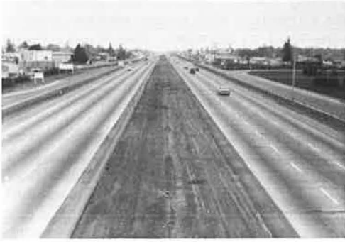
Figure 7. The Bayshore Freeway, section 17.
