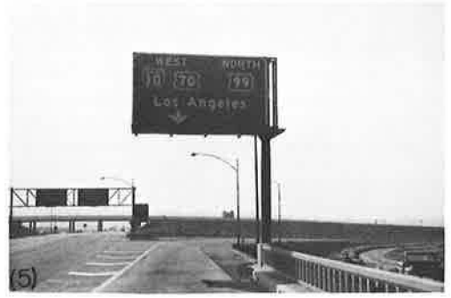
Figure 26. Construction of new ramp; southbound on US 91 to westbound on San Bernardino Freeway in Colton.
