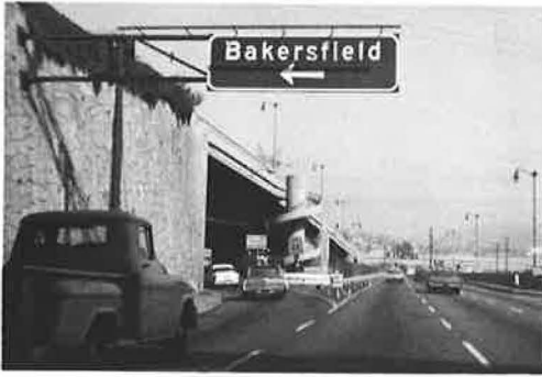
Figure 16. Eastbound on Pasadena Freeway, showing left-hand off-ramp to Golden State Freeway.
