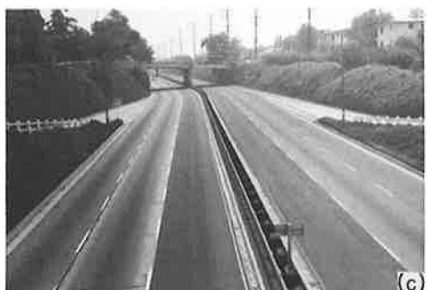
Figure 18. Section 11: (a) at Salonica Ave.; (b) southbound on-ramp at Orange Grove Ave., with stop sign; and (c) northbound on-ramp, with stop sign, and southbound off-ramp at Orange Grove Ave.
