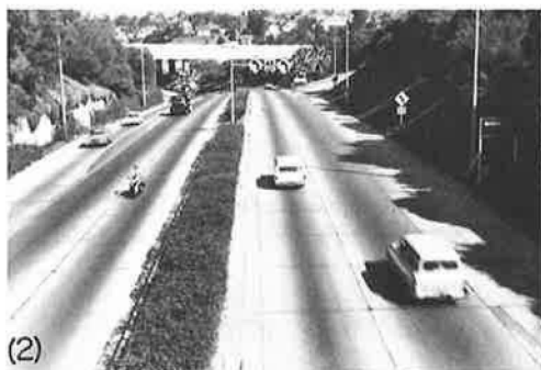
Figure 29. Washington St. interchange.
