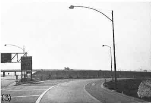
Figure 25. Drivers' view of off-ramp, southbound Rt. 43 to westbound Rt. 26.
