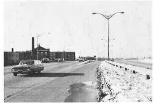
Figure 9. Diversey Ave. SB isolated left-hand entrance ramp, Kennedy Expressway, Chicago.
