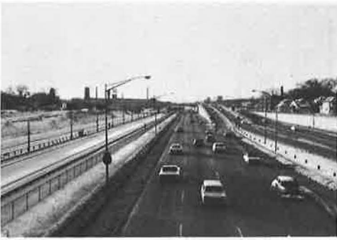
Figure 4. Harlem Ave. EB left-hand entrance ramp, Eisenhower Expressway, Chicago.
