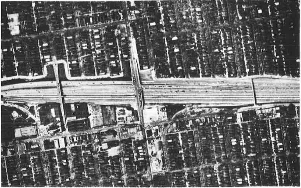
Figure 2. Aerial view of Harlem Ave. internal diamond interchange, Eisenhower Expressway, Chicago.
