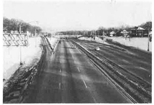
Figure 5. First Ave. WB right-hand entrance ramp, Eisenhower Expressway, Chicago.
