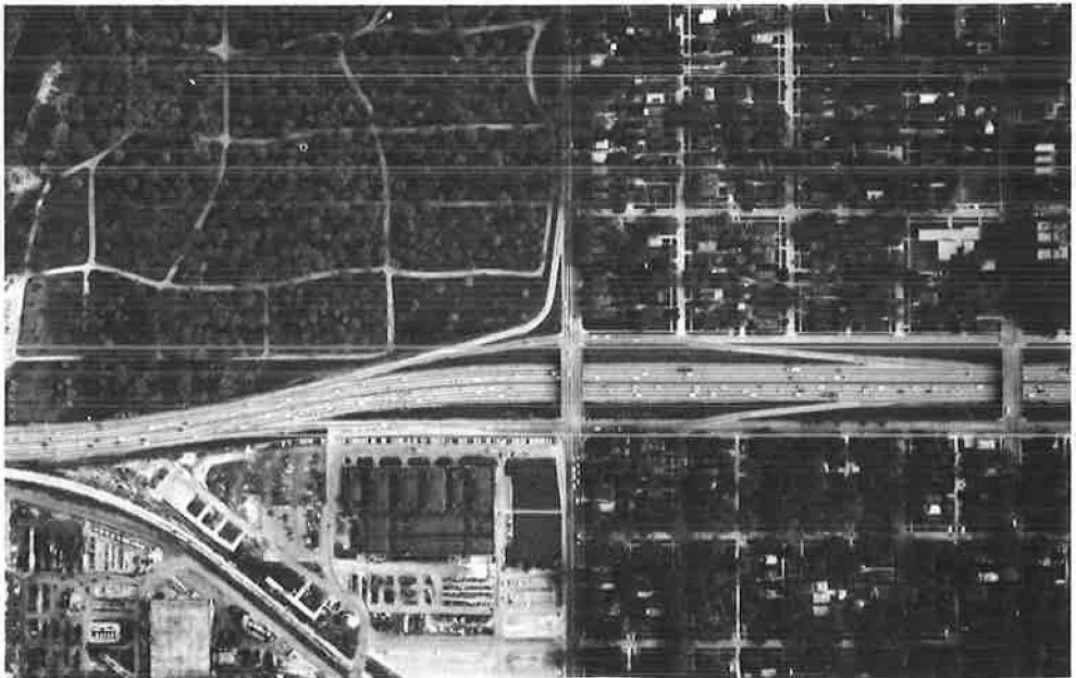
Figure 3. Aerial view of First Ave. external diamond interchange, Eisenhower Expressway, Chicago.
