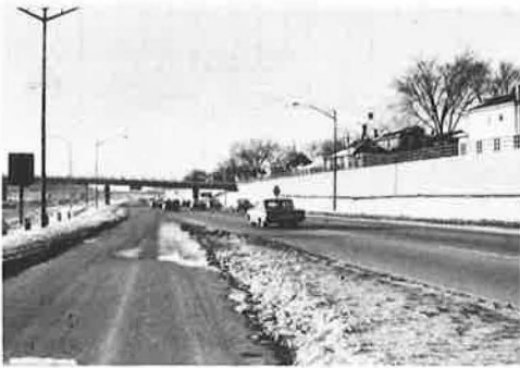
Figure 6. Austin Blvd. WB left-hand entrance ramp, Eisenhower Expressway, Chicago.
