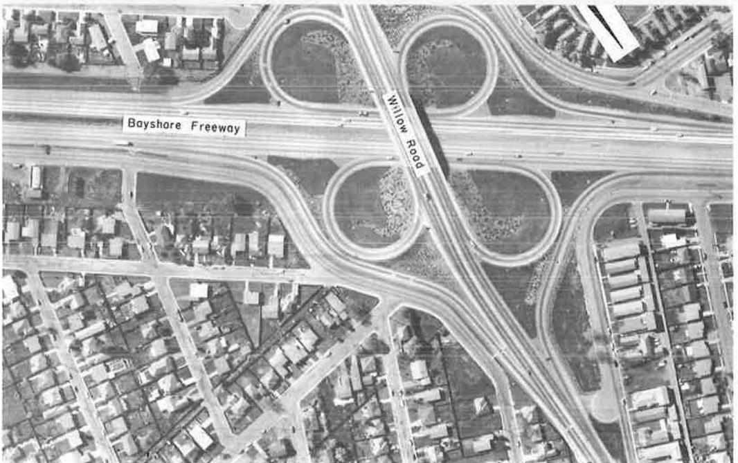
Figure 8. Willow Rd. interchange.
