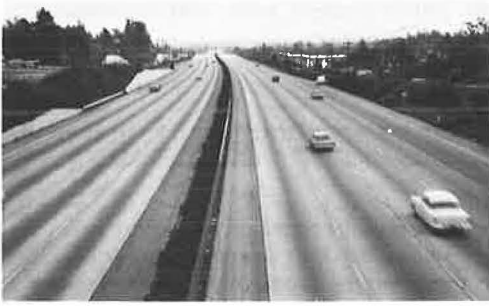
Figure 9. San Diego Freeway.
