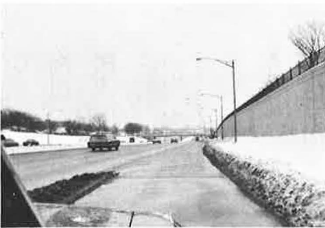
Figure 8. Sayre Ave. SB right-hand entrance ramp, Kennedy Expressway, Chicago.
