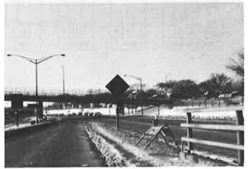
Figure 7. Harlem Ave. WB left-hand entrance ramp, Eisenhower Expressway, Chicago.
