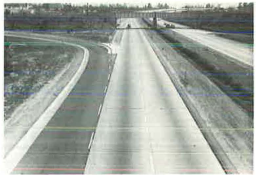
Figure 40. Hamilton Ave. interchange, southern portion.
