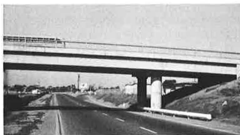
Figure 33. Off-ramp to National Ave.
