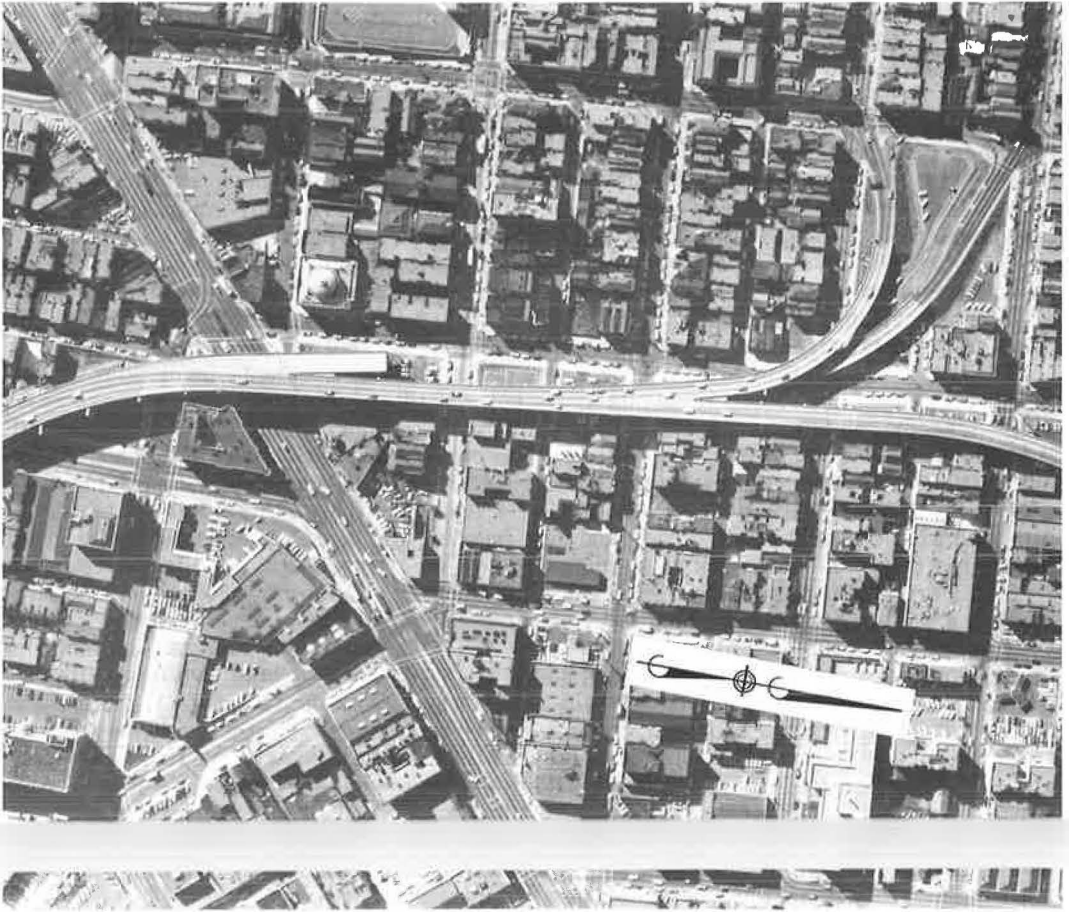
Figure 5. Central Skyway, San Francisco.
