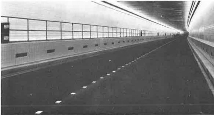
Figure 6. Two-way wedges, white non-beaded, on the roadway of the Webster Street Tube.
