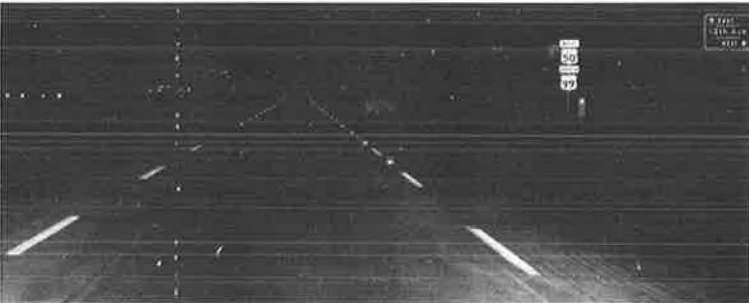
Figure 17. Reflex reflectors at night.
