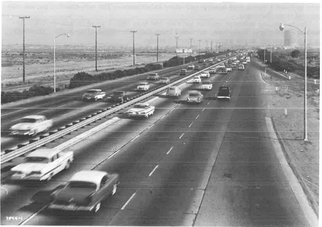
Figure 2. Double blocked-out metal beam barrier.
