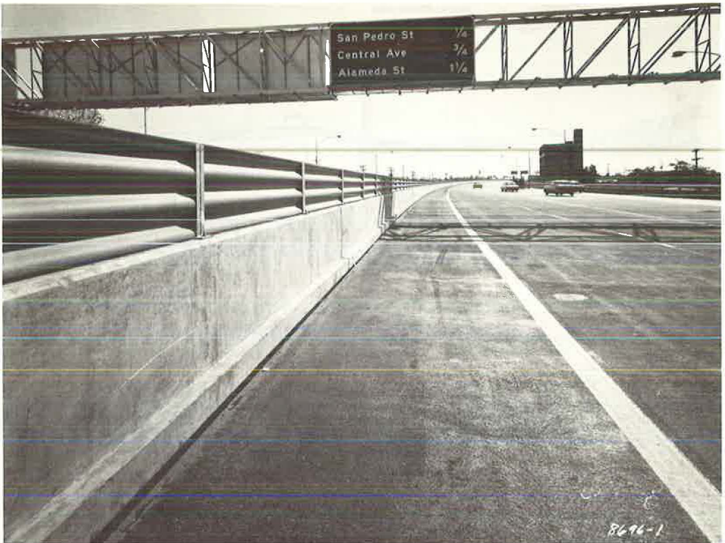
Figure 8. Concrete median barrier with headlight glare screen.
