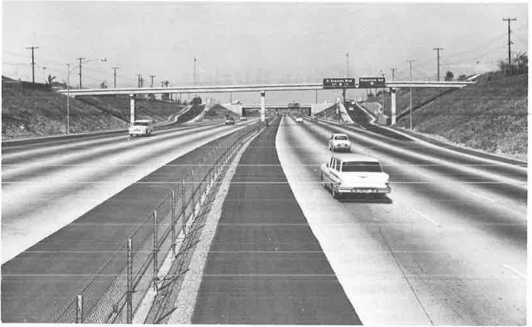
Figure 1. Cable chain link median barrier.
