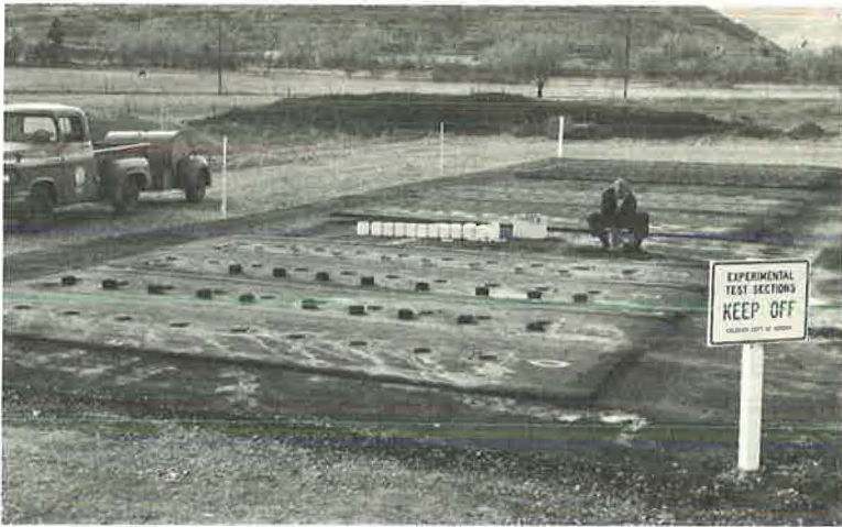
Figure 5. Coring operation on test sections completed.
