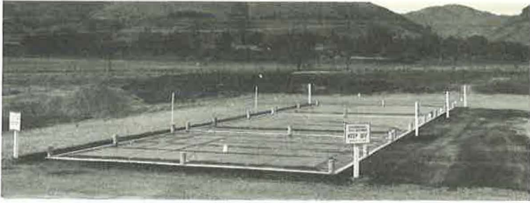
Figure 4. Polyethylene cover in place for weather protection.
