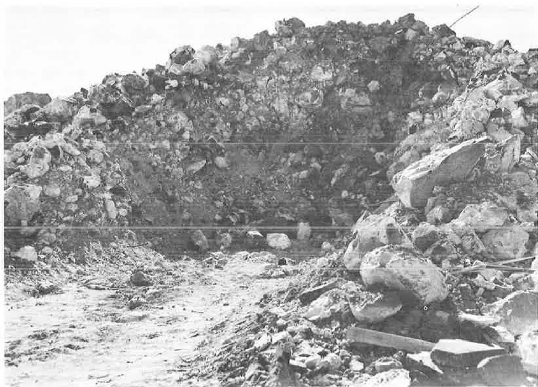
Figure 9. Trench cut partially into Sulky rubble mound, showing size distribution of rock fragments; vertical bank approximately 25 ft high.
