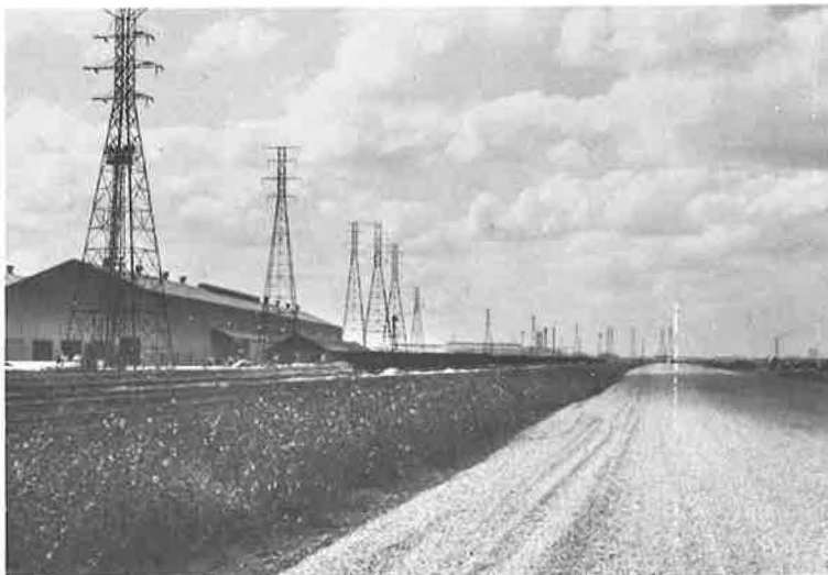
Figure 8. High-strength low-alloy steel 69-kv transmission towers, Gary Steel Works.
