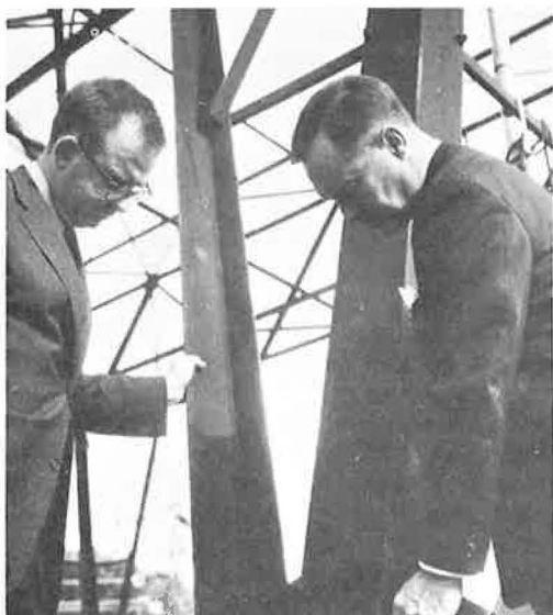
Figure 9. Appearance of high-strength low-alloy steel in Project EHV after 2 yr near Pittsfield, Mass.
