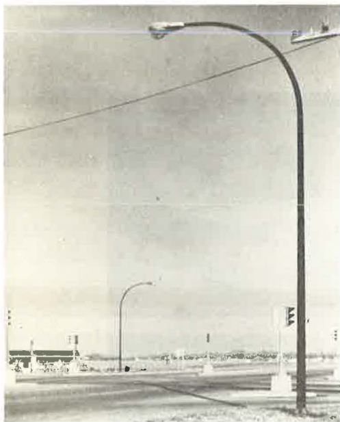
Figure 18. High-strength low-alloy steel light standards in midwestern city.
