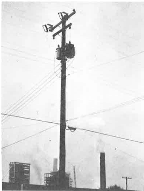
Figure 12. Effluent from smoke stack deposits on transformer tank of high-strength low-alloy steel and painted carbon steel, Georgetown, S.C.
