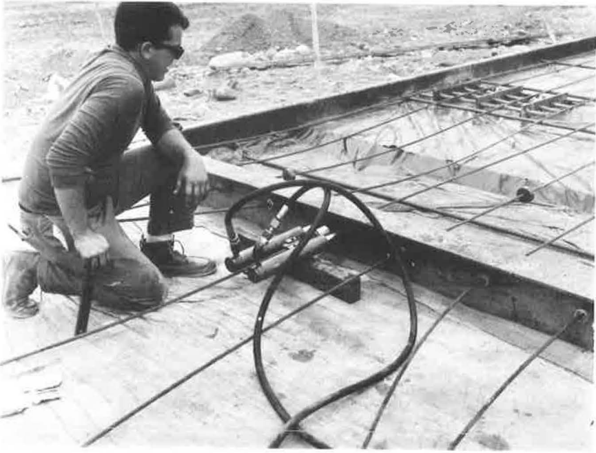
Figure 10. Tensioning of longitudinal prestressing reinforcement cables.
