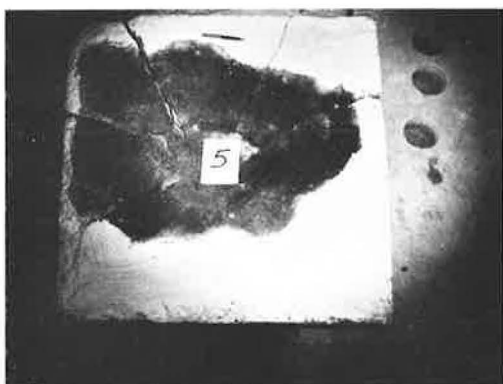
Figure 19. Bottom face of inverted section of pavement after failure under static load.
