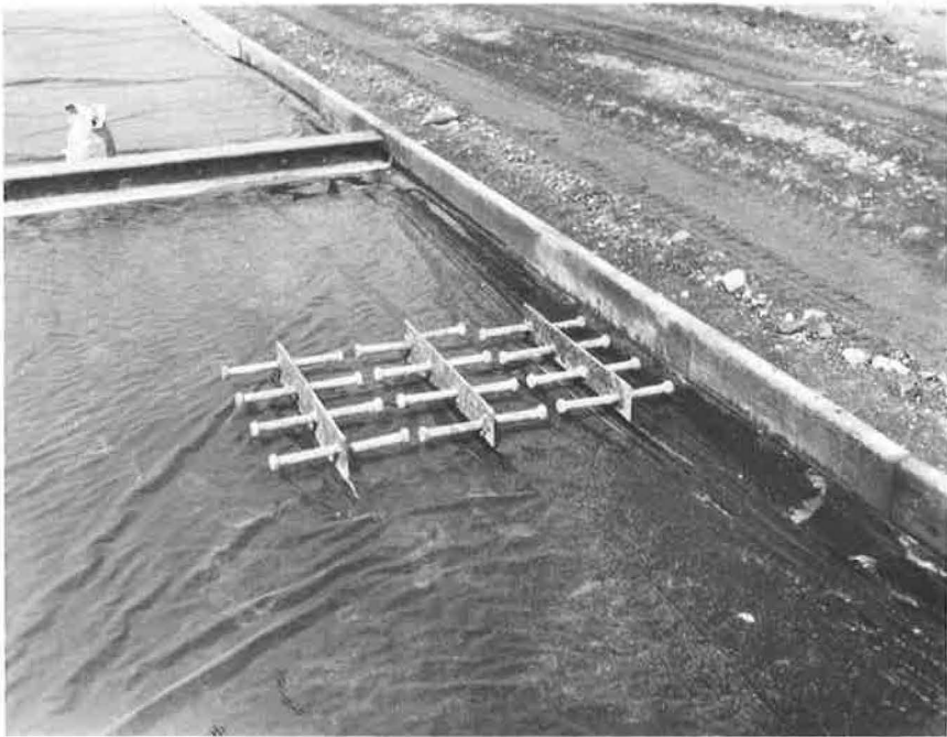
Figure 9. Polyethylene sheeting being carried over surface of sleeper slab.
