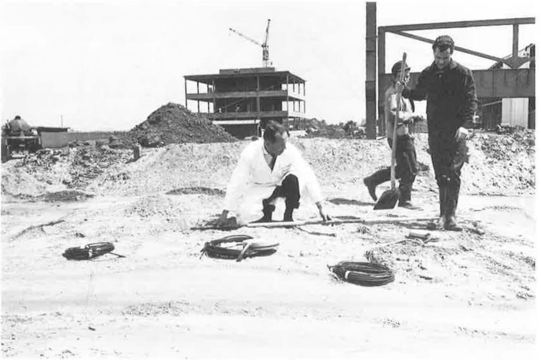
Figure 22. Installing Heierli pressure cells.
