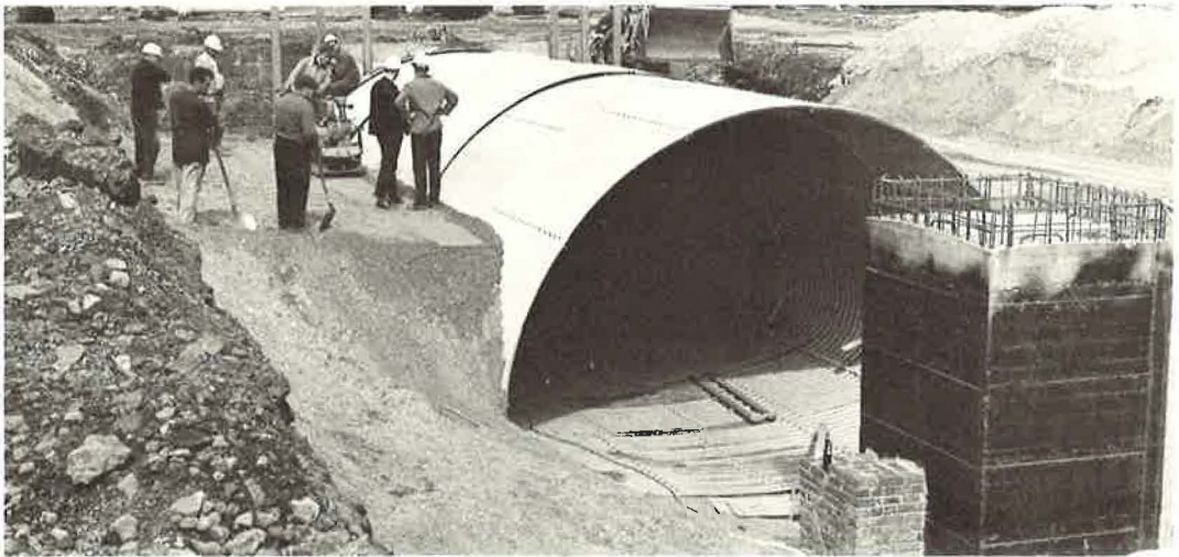
Figure 2. Placement and compaction of backfill.
