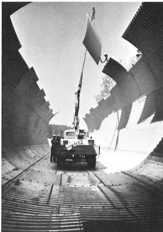
Figure 44. Special profile S 32 during construction.
