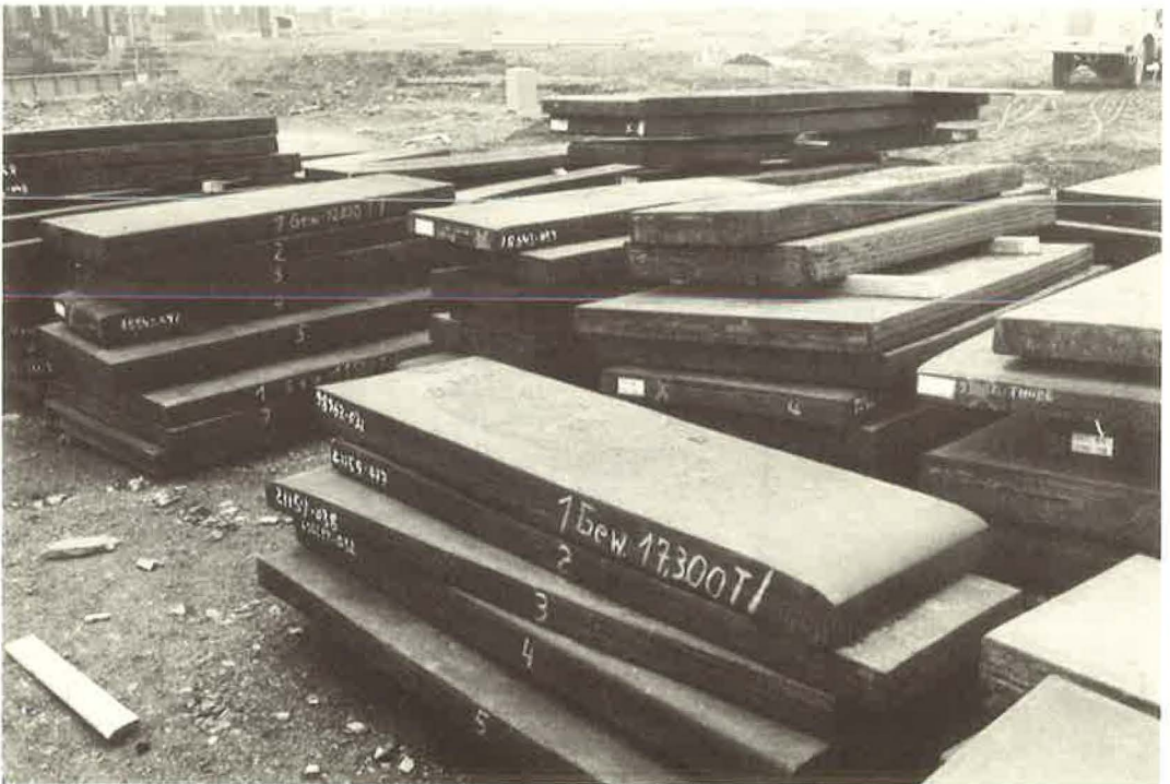
Figure 7. Slabs ready to be placed on structure.
