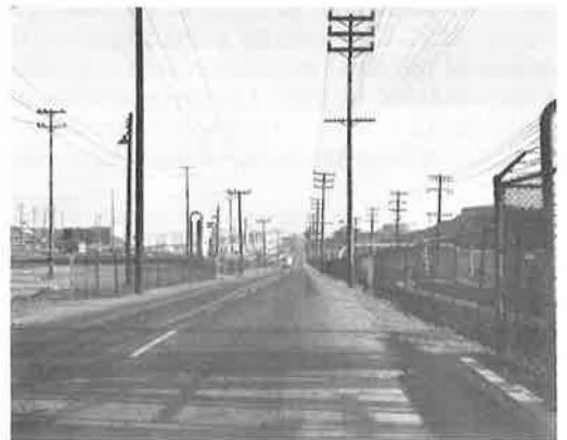
Figure 3. General view of test road, after resurfacing.
