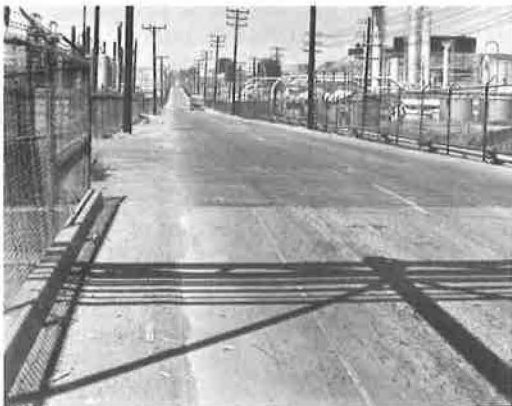
Figure 2. General view of test road, before resurfacing.
