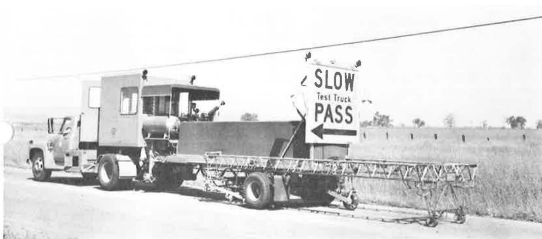
Figure 1. Traveling deflectometer.
