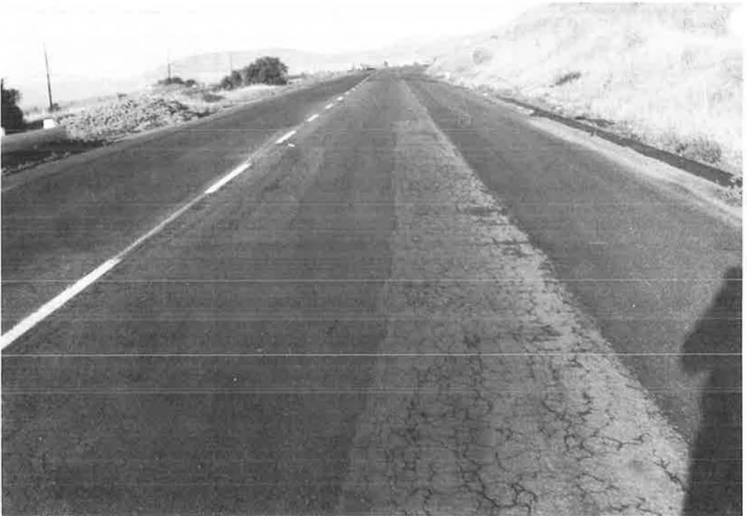
Figure 5. Road V-SLO-2-PBch, E, northbound travel lane.
