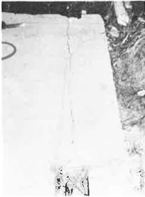
Figure 5. Failure at slot J.
