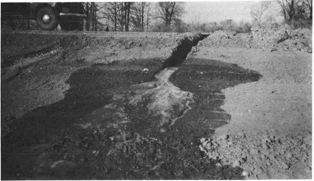
Figure 4. Drainage of subgrade on US 301, fall 1955.
