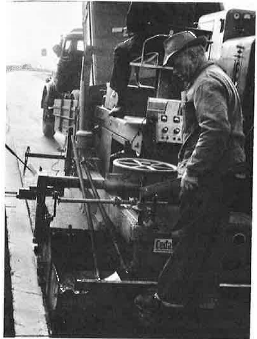
Figure 6. Automatic screed control paver, showing control panel.
