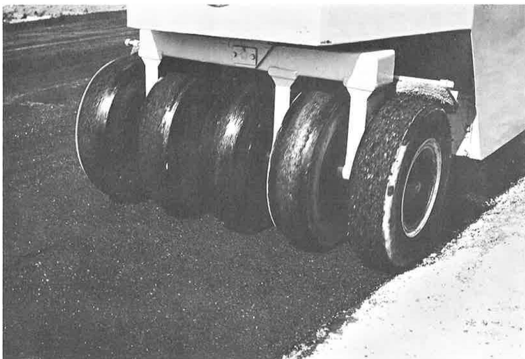
Figure 2. Mix sticks at moderate temperature (160 F) to pneumatic tires lubricated with water.
