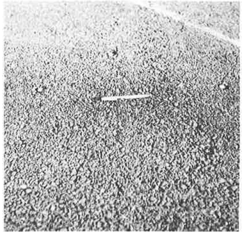
Figure 26. Right wheel tracks at cross-over at 46 hr (5,330 trips).
