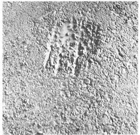
Figure 6. Test no. 12 (two runs of studded tire side-by-side, on new asphaltic-concrete shoulder): scour, 9.0 x 0.64 in. deep; breakout of intervening pavement.
