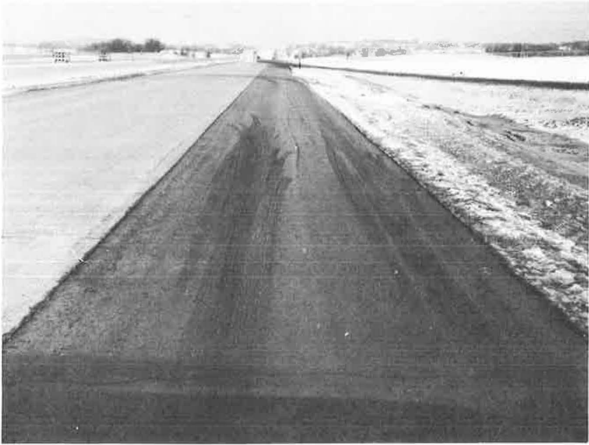
Figure 9. Bituminous surface after 210 panic stops.
