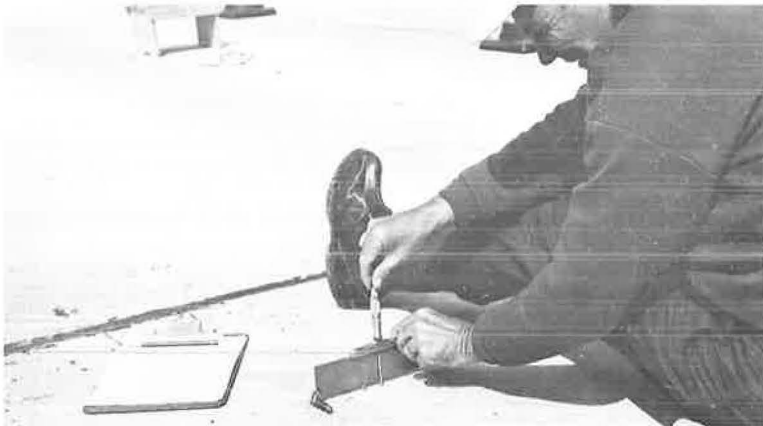
Figure 6. Depth gage, Vernier method.
