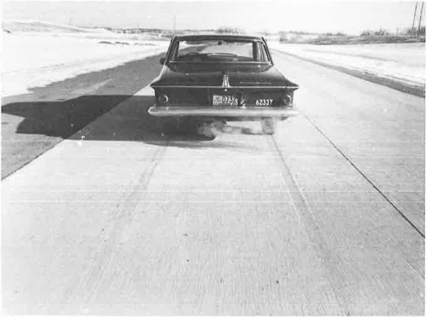
Figure 5. Concrete surface after single panic stop.
