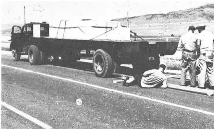
Figure 7. Benkelman beam deflection test.
