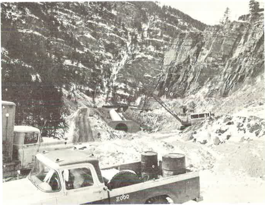
Figure 3. Inlet end of culvert during construction.
