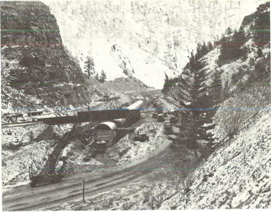
Figure 2. Outlet end of culvert during construction.
