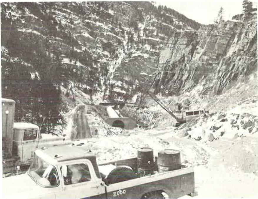
Figure 3. Inlet end of culvert during construction.
