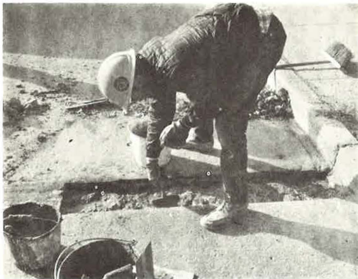
Figure 6. Applying brush coat of epoxy adhesive.
