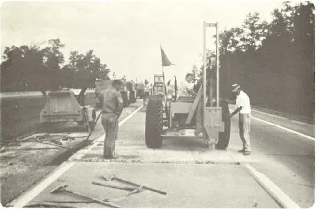
Figure 6. Drop hammer breaking out 2- by 3-ft concrete pieces.
