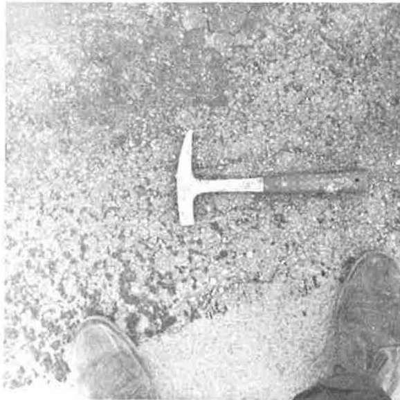
Figure 5. Test panel No. 9, showing slight reflection cracking.
