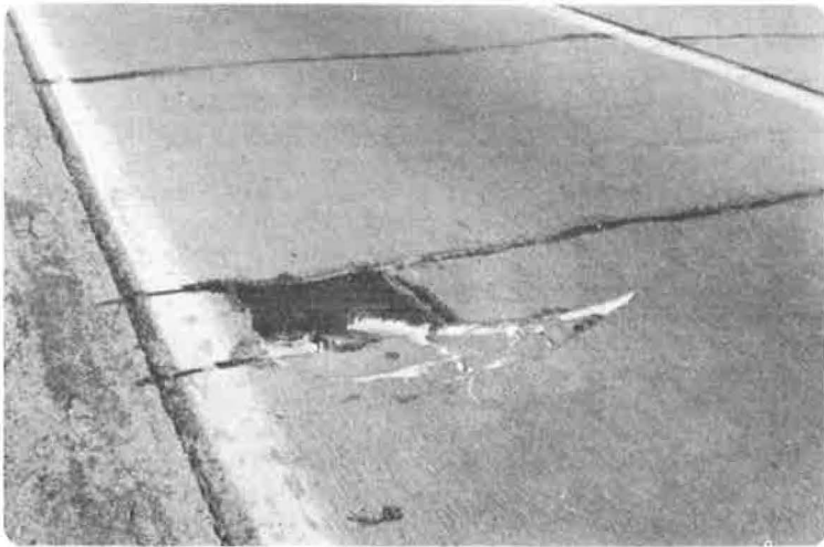
Figure 1. Patch design and position in pavement with respect to joints and edges.
