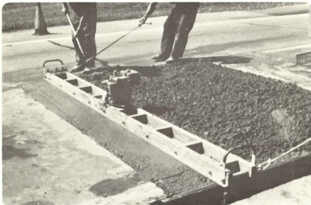
Figure 14. Addition of remaining concrete after placement of steel mesh.
