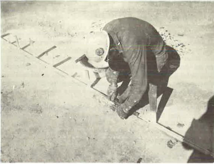
Figure 7. Placing wooden form.
