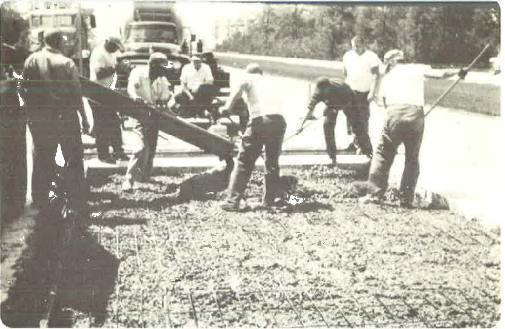
Figure 11. Placement of ready-mix concrete.
