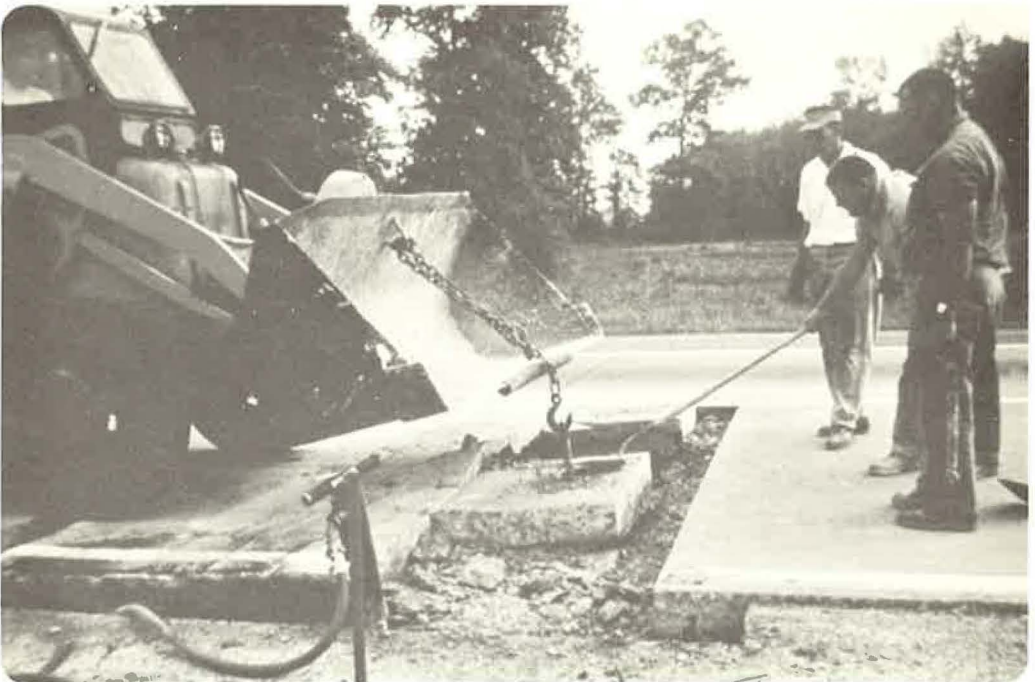
Figure 7. High-lift used to lift out piece of slab.
