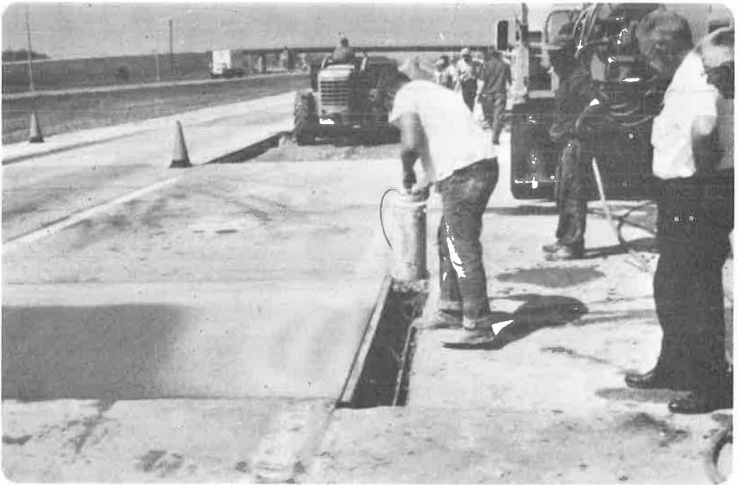
Figure 15. Spraying of white-pigmented compound on concrete.
