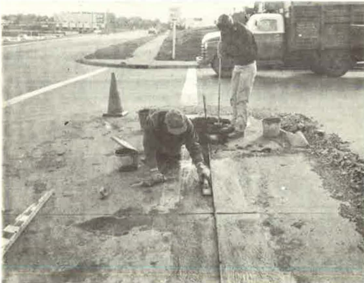
Figure 8. Tamping mortar into patch.
