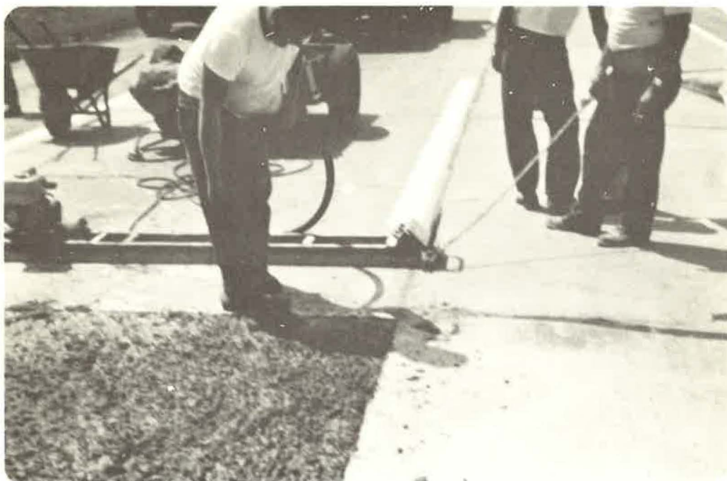
Figure 13. Placing of concrete in repair area.
