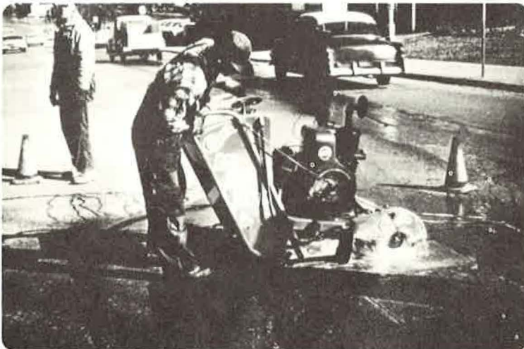
Figure 3. Sawing of pavement to cut reinforcing steel.
