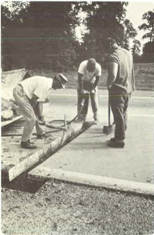
Figure 5. Trench in shoulder beside slab to accommodate forms.
