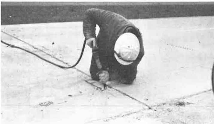
Figure 5. Using a small chipping hammer in small, shallow areas.
