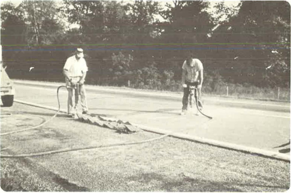
Figure 4. Drilling of hole for lift pin which removes concrete piece.
