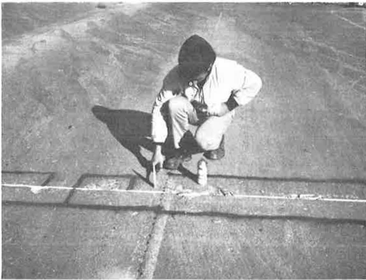
Figure 4. Painting outline of unsound concrete.
