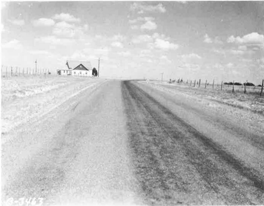
Figure 56. No center stripe concentrates traffic in center third of FM 1192.
