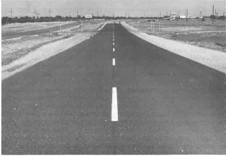
Figure 48. Type F seal two years old with 7700 vpd.
