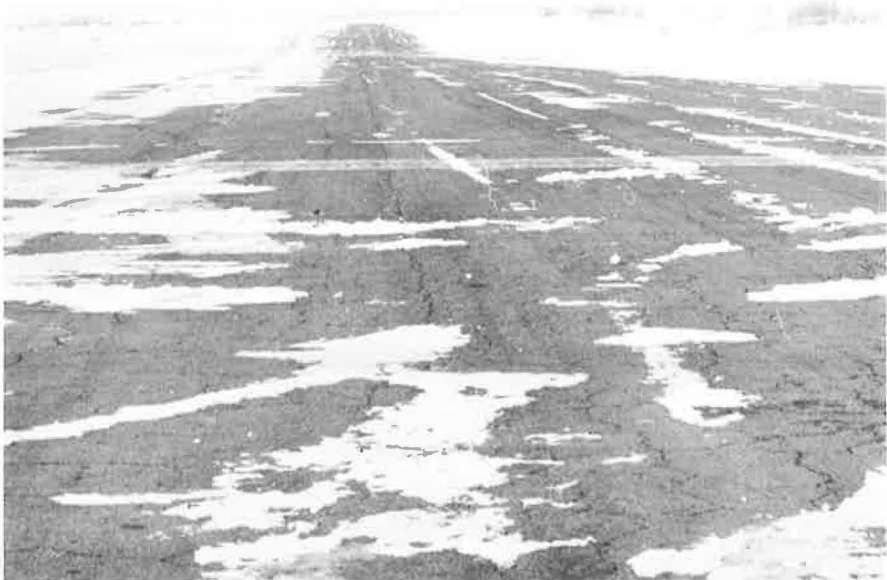
Figure 3. Caribou runway before bituminous macadam overlay.
