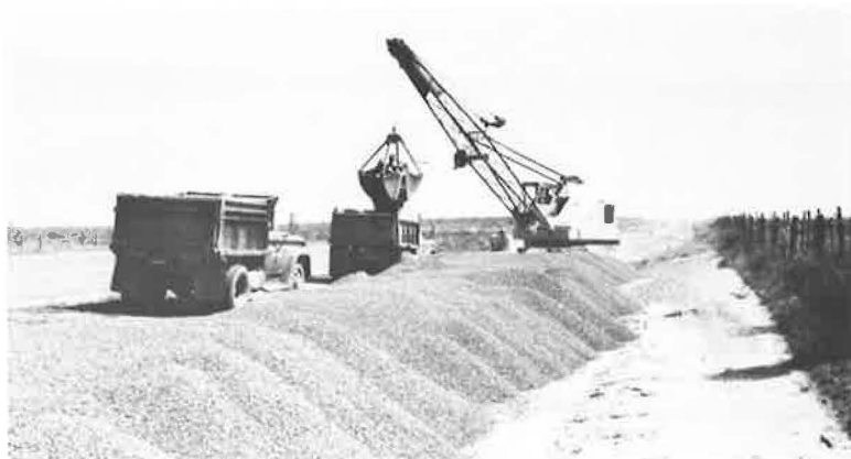
Figure 50. Stockpile and loading operation of type F material.
