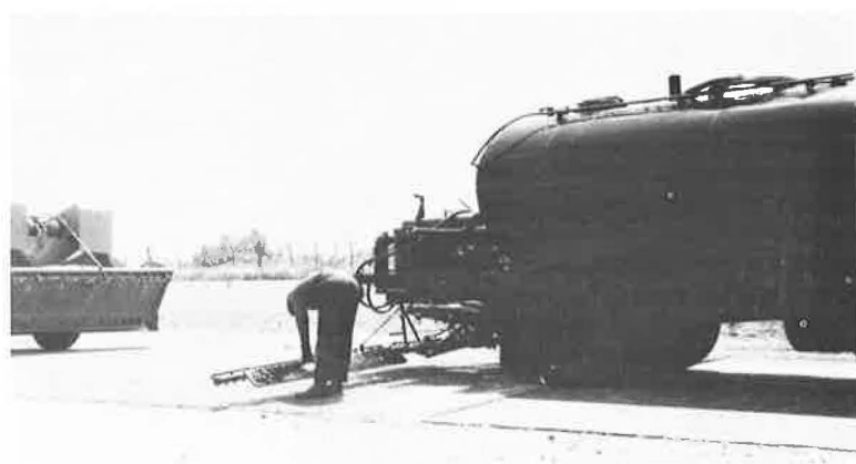
Figure 51. Distributor operator placing wind guard on spray bar.
