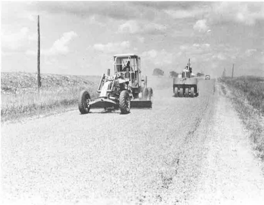
Figure 61. Blade broom successfully used on type F coverstone.
