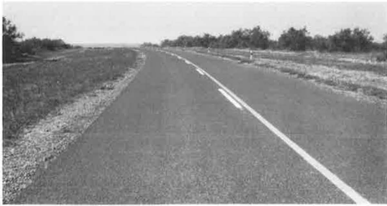
Figure 54. Type F material after one year of light traffic.
