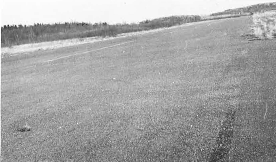
Figure 2. Eastport Airport after a 3-in. bituminous macadam overlay.
