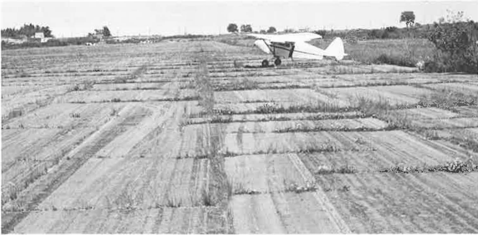
Figure 1. Eastport Airport before bituminous macadam overlay.
