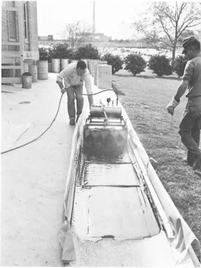
Figure 12. Hot asphalt cement being sprayed from small distributor.
