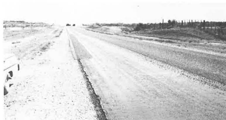
Figure 52. Patches create variations in asphalt demand of surface.
