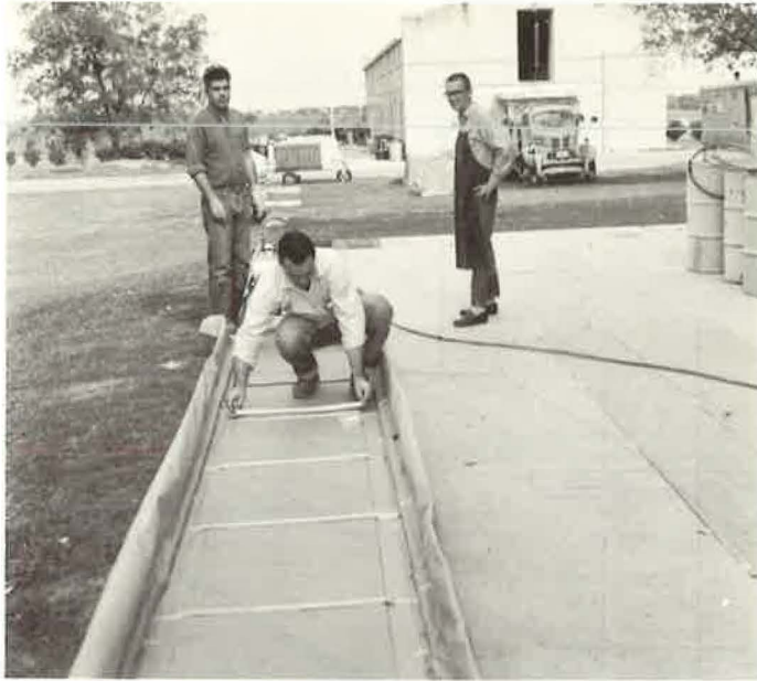
Figure 10. Boards in line for asphalt shot.
