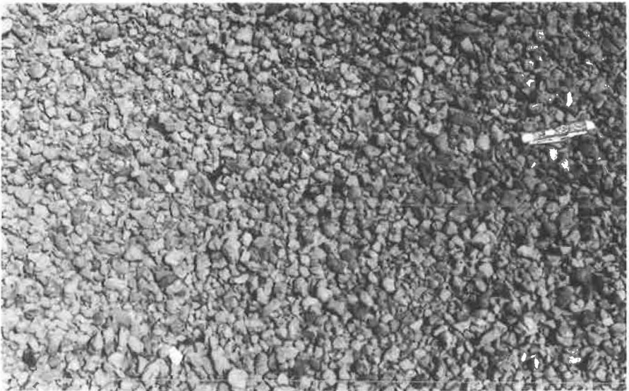
Figure 63. Type F Grade 3 after brooming. Spread rate—130 sq yd/cu yd.
