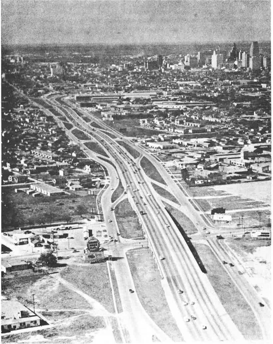
Figure 3. Gulf Freeway, Houston, Texas.
