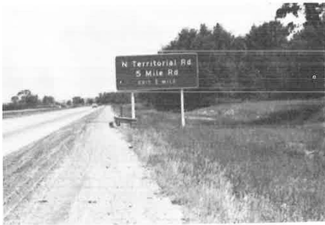
Figure 26. Expressway sign with support completely unprotected by guardrail.
