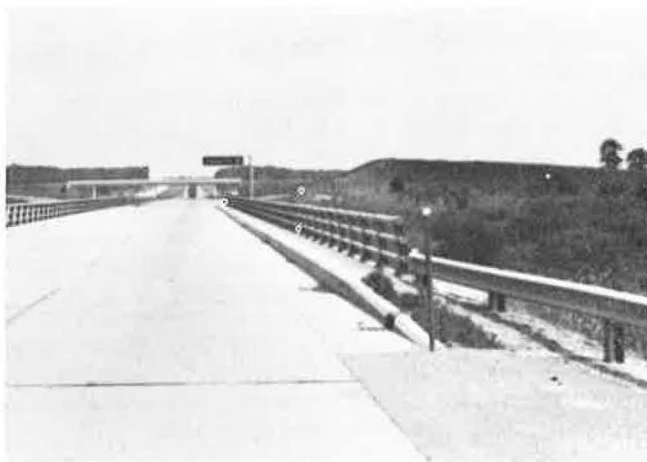
Figure 28. Typical bridge rail design with sidewalk.
