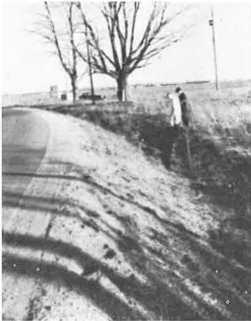
Figure 6. Deep ditch adjacent to road. Vehicle traversed ditch, flew 50 ft and impacted the roof, hood, and trunk against tree located 31 ft from roadside.
