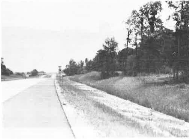
Figure 24. Deep drainage ditch near expressway.
