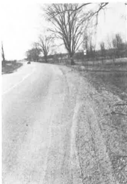
Figure 2. Vehicle left roadway on right side of curve and struck tree (center) 15 ft from edge of road. Driver killed.
