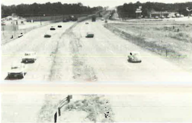
Figure 16. Narrow (27 ft) median allowing flat bed trailer to cross and strike a car.
