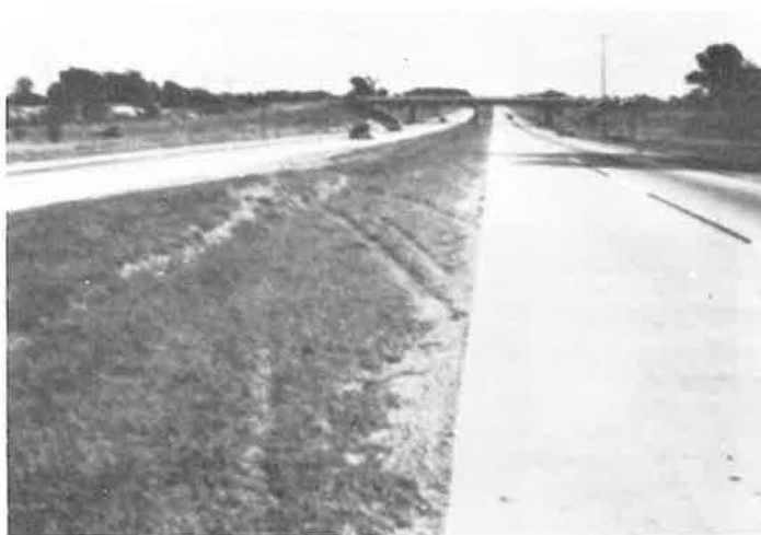
Figure 14. Narrow (26 ft) median at point of crossover. Vehicle hit drainage ditch in center of median, rolled over striking another car.
