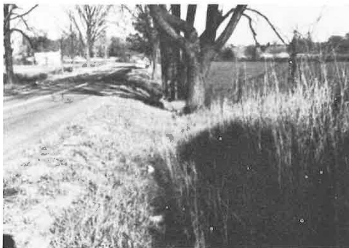
Figure 10. Steep slope prevented return of car to roadway before impact. Trees are 25 ft from road edge.
