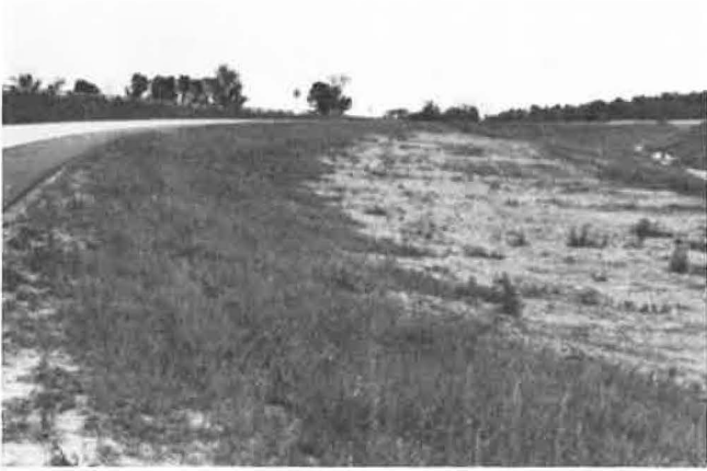
Figure 21. Expressway entrance ramp. Note obstacle clear, off-road area.
