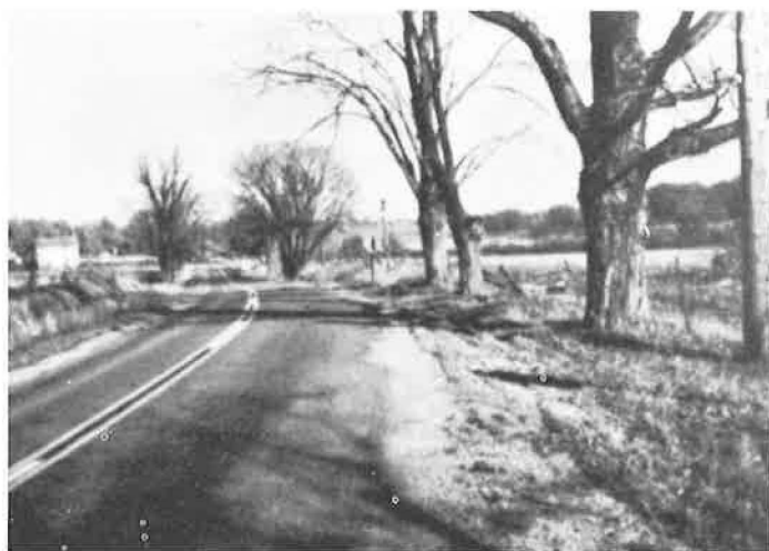
Figure 9. Entrapment of vehicle by drainage ditch next to embankment led it to distant trees. Ditch 10 ft from roadside.
