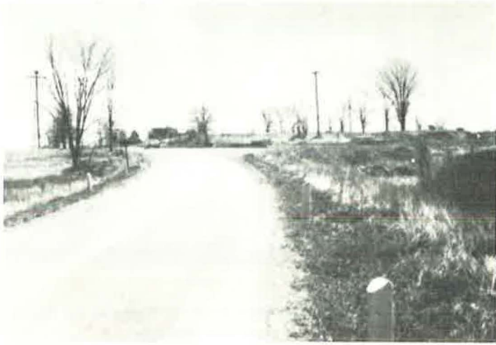
Figure 7. Vehicle "missed the curve" knocking down several guard posts and hit earth embankment in the distance. Proper guardrail design would have prevented a straight-on course to embankment which should have been removed. Impact point location 20 ft from road edge.
