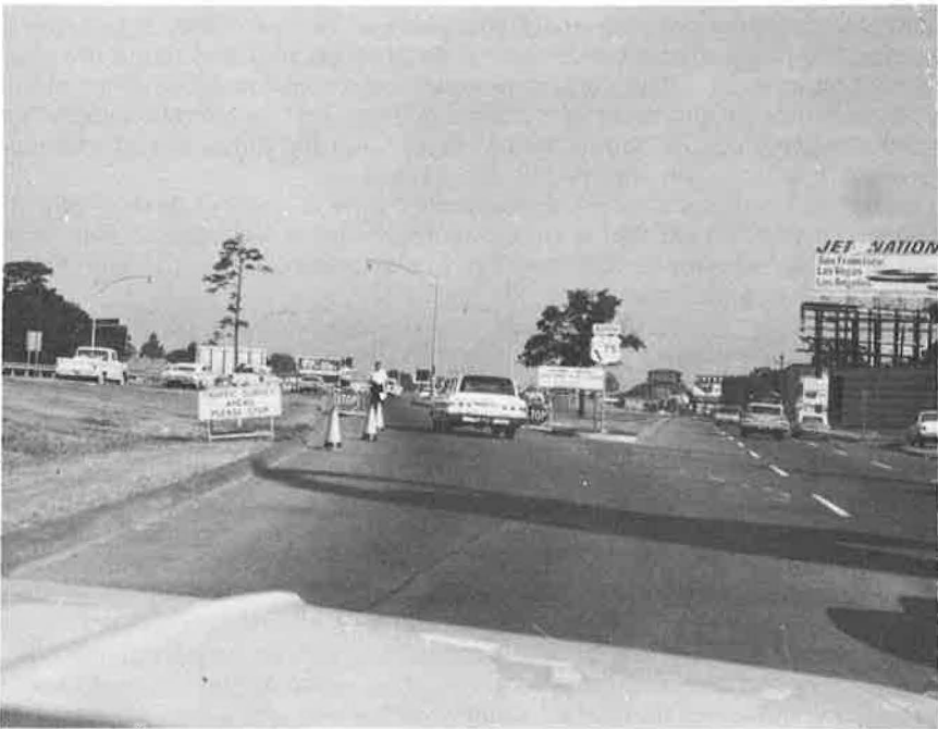
Figure 7. Ramp metering location.
