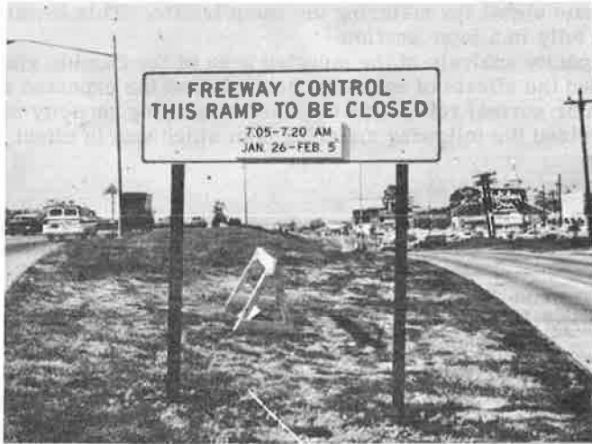
Figure 3. Advisory signs erected at ramps to be controlled.
