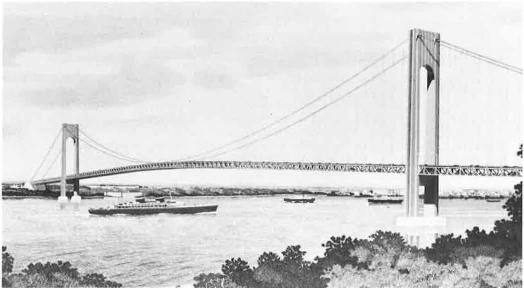
Figure 1. General view of Narrows Bridge.
