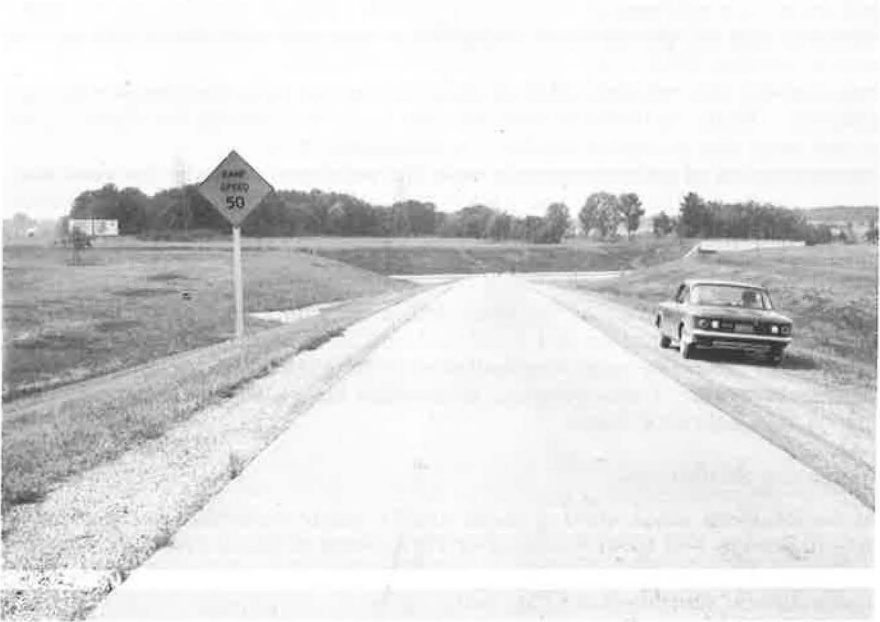
Figure 21. Westbound entrance ramp to 174 near Danville, Illinois.
