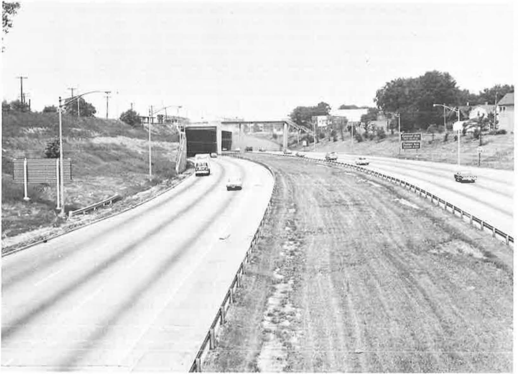
Figure 6. View of Kennedy Expressway showing reserved median.
