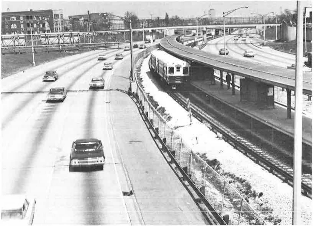
Figure 5. View of Congress rapid transit facility.
