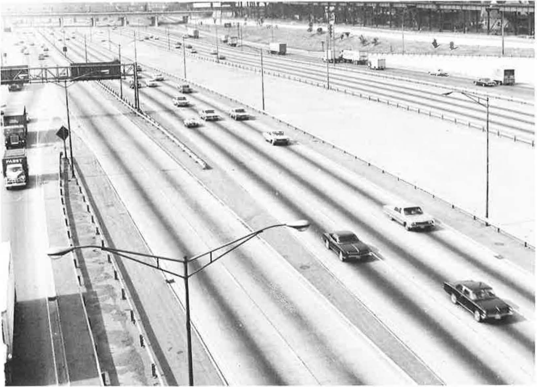
Figure 7. View of Dan Ryan Expressway showing reserved median.
