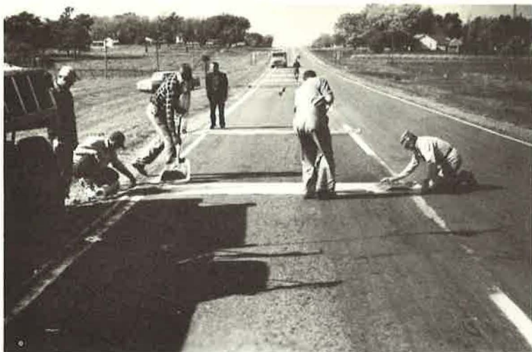
Figure 8. Approach A 1 , placing paper prior to the application of RS-3K.
