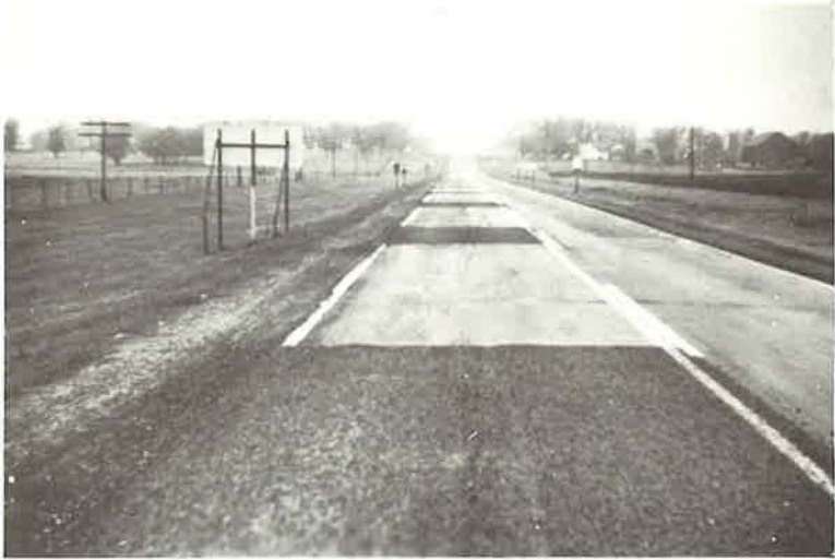
Figure 4. Approach A 1 , looking west.
