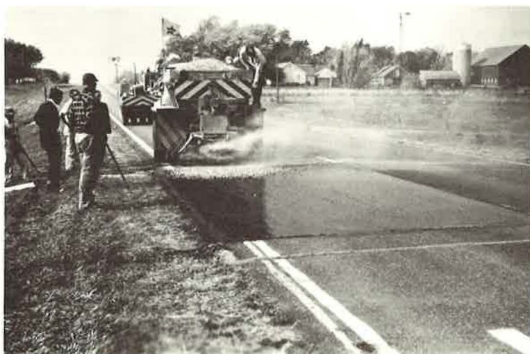
Figure 9. Approach A 1 , spreading aggregate.
