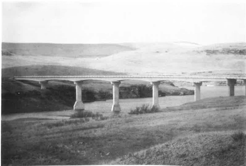
Figure 29. Another view—a graceful bridge until we look far right.
