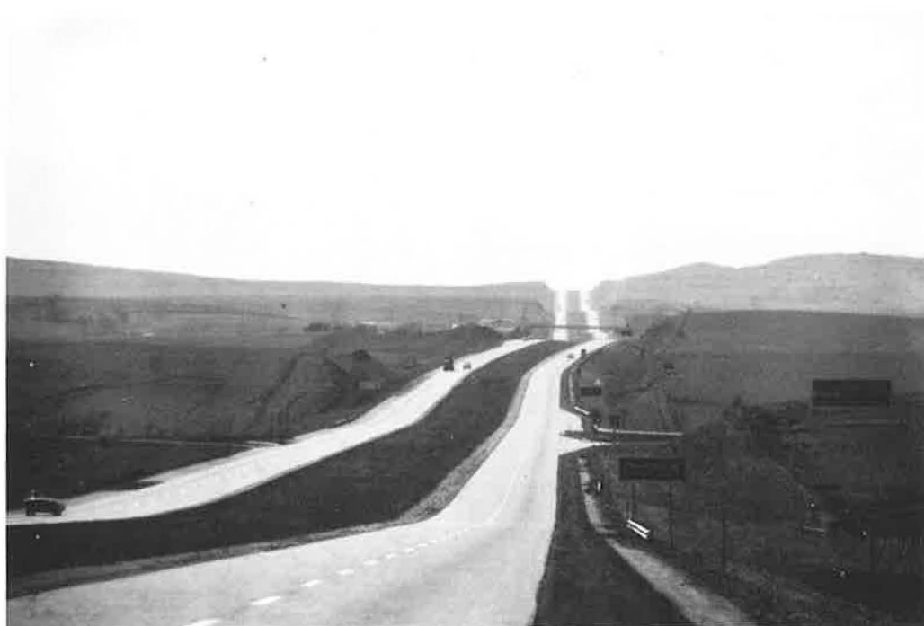
Figure 24. More common: the broken-back with small grade changes. This type of design destroys the flowing continuity of a high speed highway. Note the jerk in horizontal alignment.
