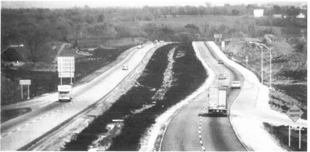
Figure 1. To appreciate more fully the value of good design it is instructive to observe a few examples of discontinuous alignment where "how it looks" was considered unimportant. A continuous curve beginning at the bottom of the slide and ending where the right lane disappears would have been a much superior design.
