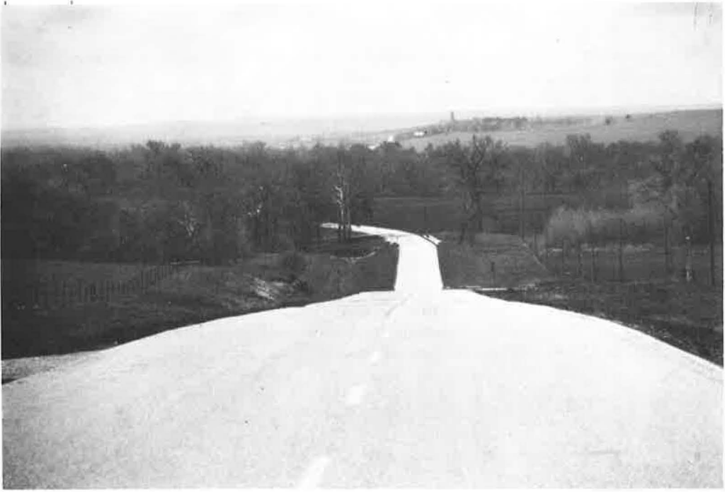
Figure 35. The view is shortened and we're looking into a wide pleasant valley. The road ahead points to the left for driver guidance. Perhaps a longer vertical curve would have made this view even more pleasing.
