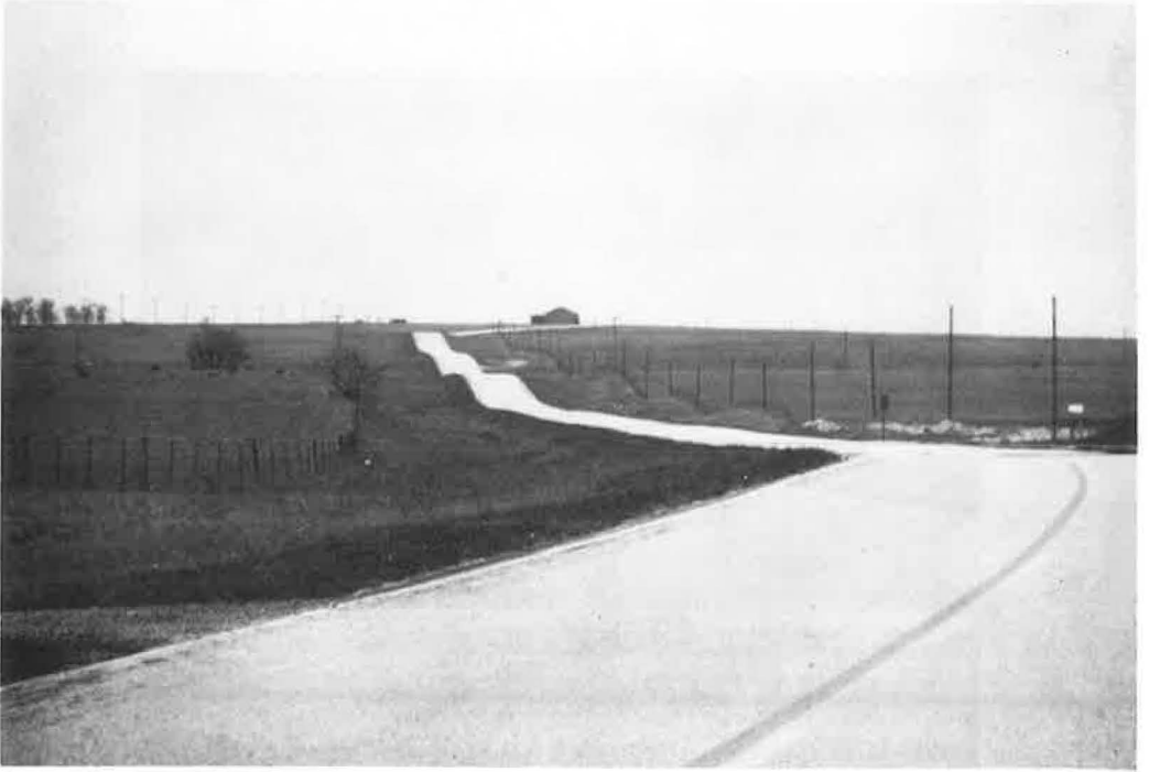
Figure 5. The Blue Book (7) states, "The 'roller-coaster' or the 'hidden-dip' type of profile should be avoided. Such profiles generally occur on relatively straight horizontal alignment where the roadway profile closely follows a rolling natural ground line. They are unpleasant aesthetically and hazardous."
