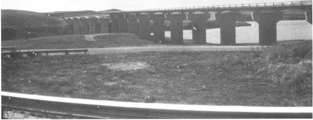
Figure 31. By changing from one type of bridge construction to another, the number of piers was nearly doubled—the continuity of this design was lost (8). Also lost was the opportunity to provide a striking picture of civil engineering creativity for the thousands of reservoir visitors who will pass under this bridge and view it from near and from afar.
