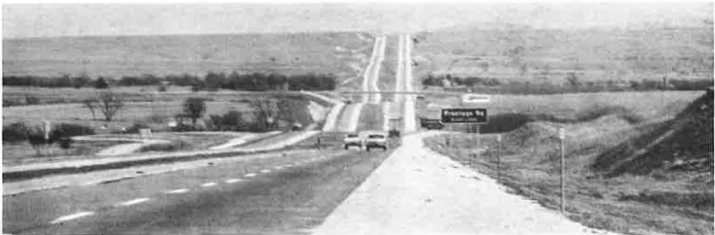
Figure 4. Because of straight alignment one often can see a long distance ahead. When this happens it is almost impossible to avoid a roller-coaster appearance. Secondly, any median width changes are difficult to conceal. Observe the width change just above the grade separation structure.
