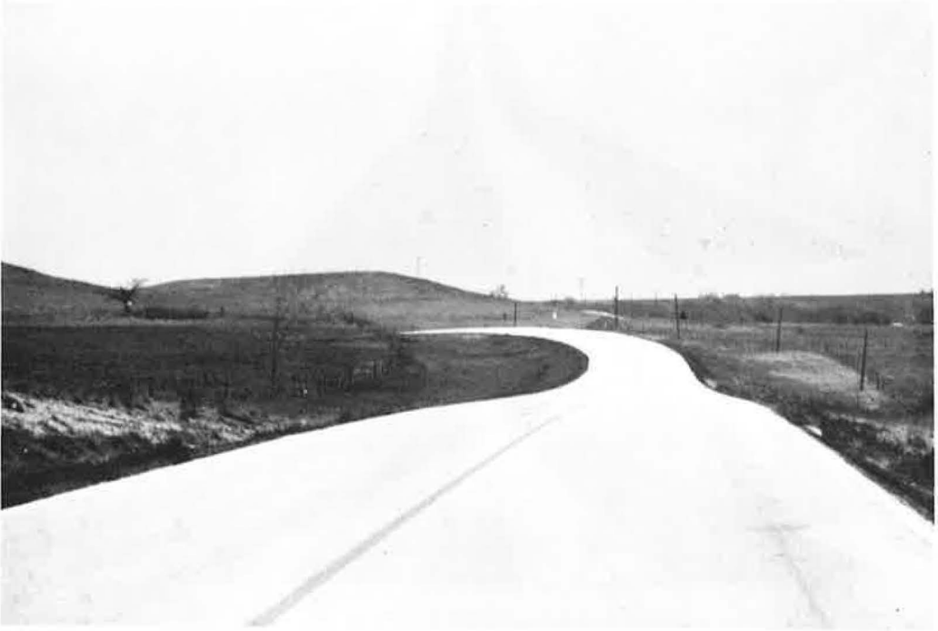
Figure 15. A short vertical curve at the beginning of a horizontal curve. Again, this is not a well-balanced design.
