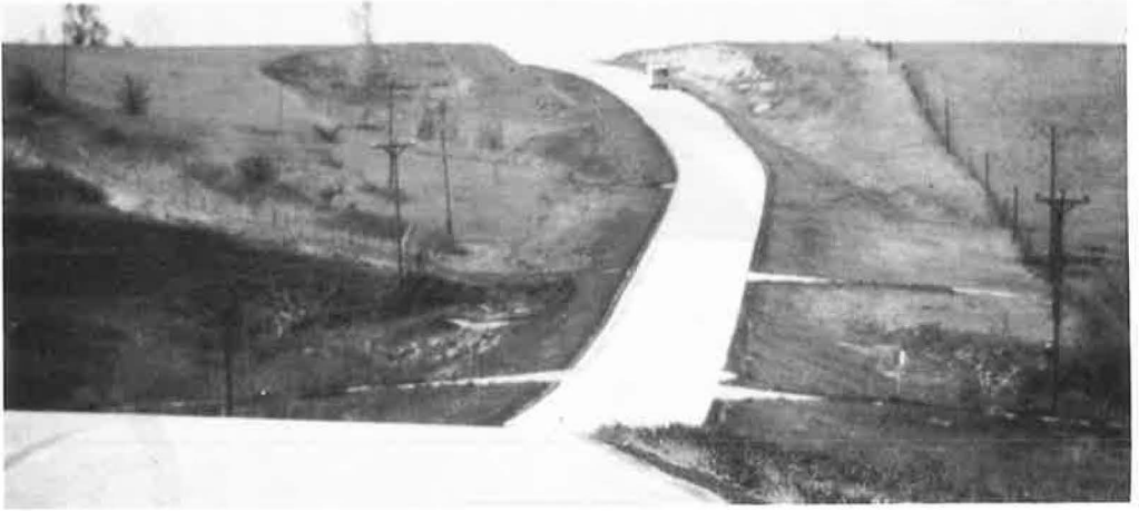
Figure 13. A long spiral beginning at the first entrance at the bottom of the hill and ending near the position of the truck would have improved the appearance of this curve.
