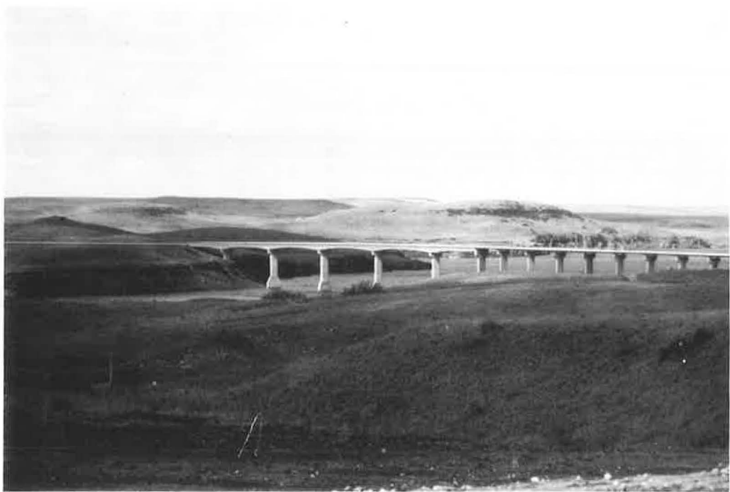
Figure 30. There appears to be little reason for changing to the concrete bridge on the right.
