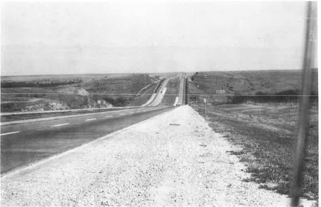
Figure 18. The curve at the bottom of the hill is too short when viewed from this distance.
