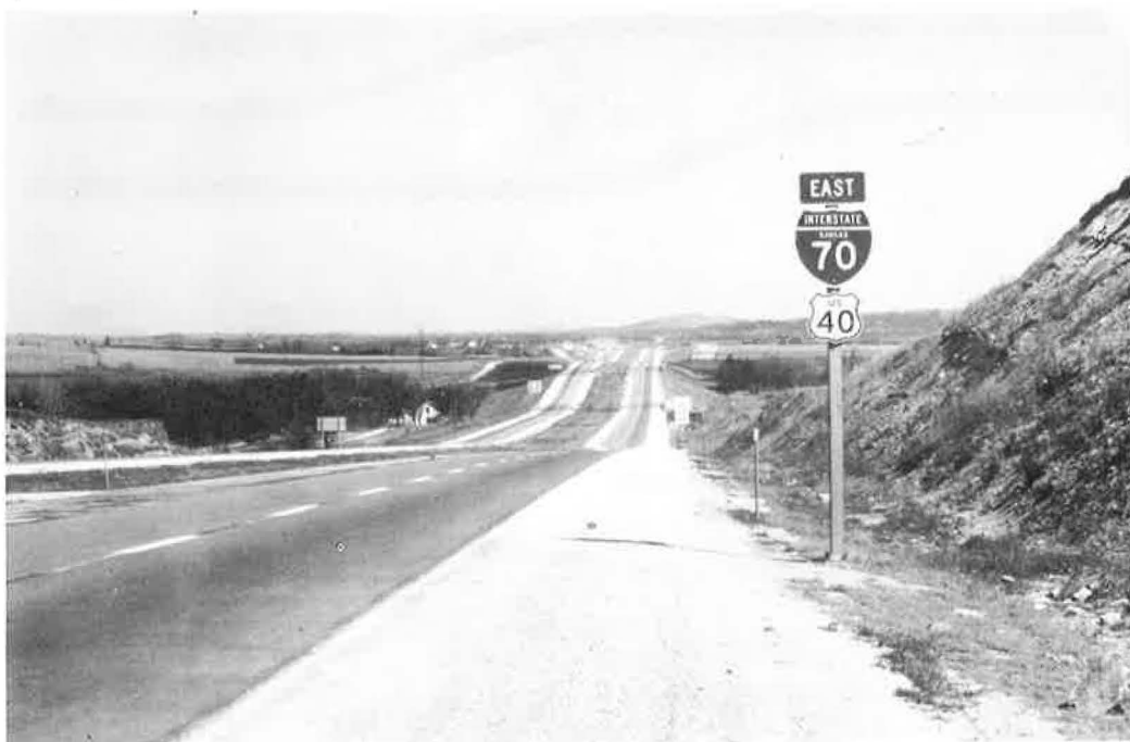
Figure 23. A "broken-back" vertical alignment.
