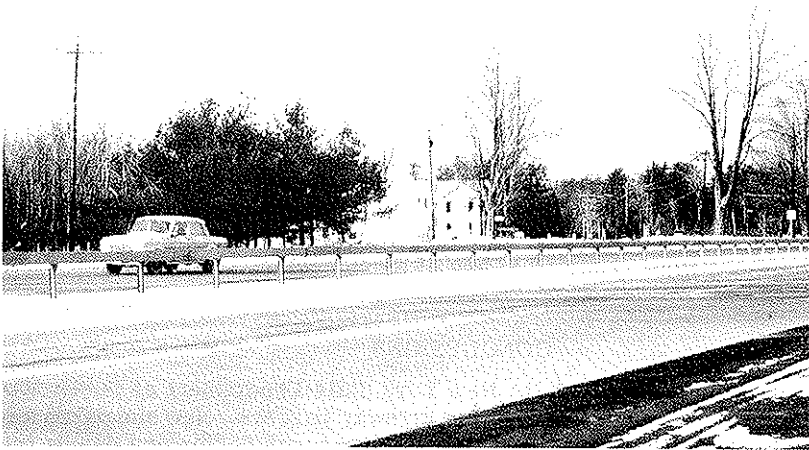
Figure 89. Box beam median barrier.
