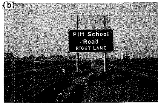
Figure 9. (a) Possible location for back-to-back signs; (b) back-to-back signs.
