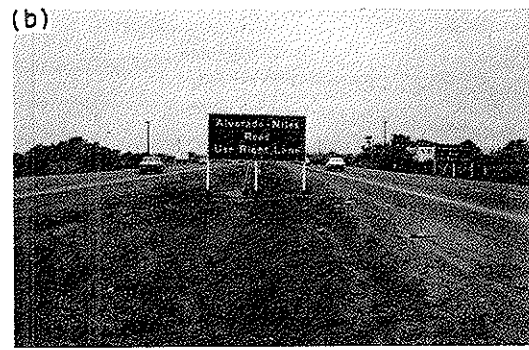
Figure 16. (a) Sign with steel posts which could have been placed on timber posts; (b) sign on timber posts.
