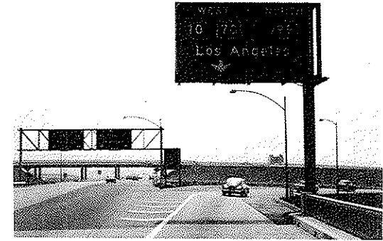
Figure 13. Signpost placed immediately beyond bridge rail.
