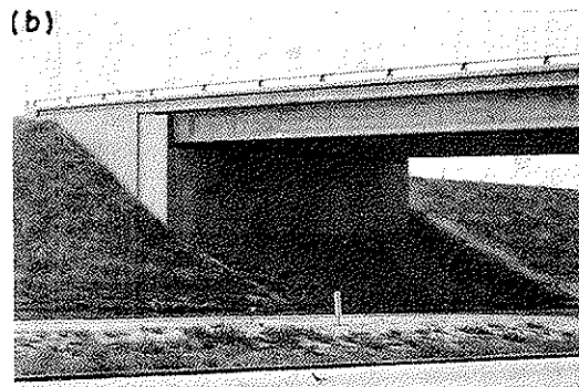
Figure 7. (a) Possible location for enclosing side abutment in fill cone; (b) side abutment enclosed in fill cone or cut slope.
