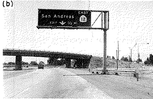
Figure 12. (a) Gore sign could be replaced by overhead sign adjacent to right shoulder at beginning of ramp taper and a structure-mounted sign for next exit; (b) overhead sign adjacent to shoulder.
