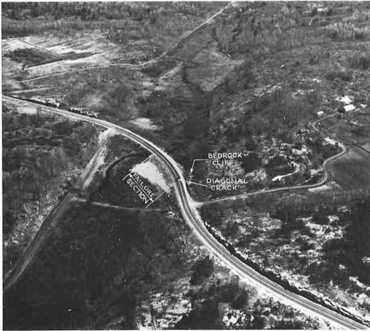
Figure 2. Site and embankment after repairs.
