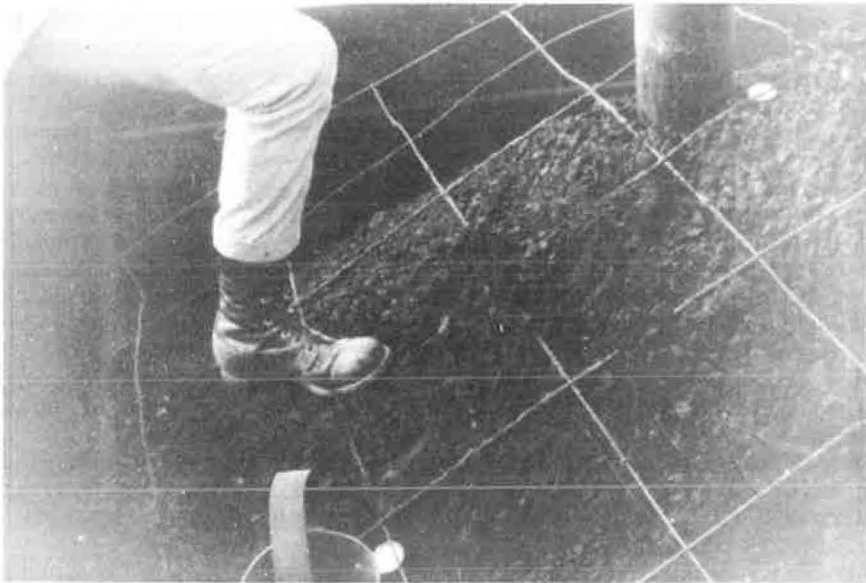
Figure 2. Sampling mix from batch truck, showing grid, sampling device, and thermometers.
