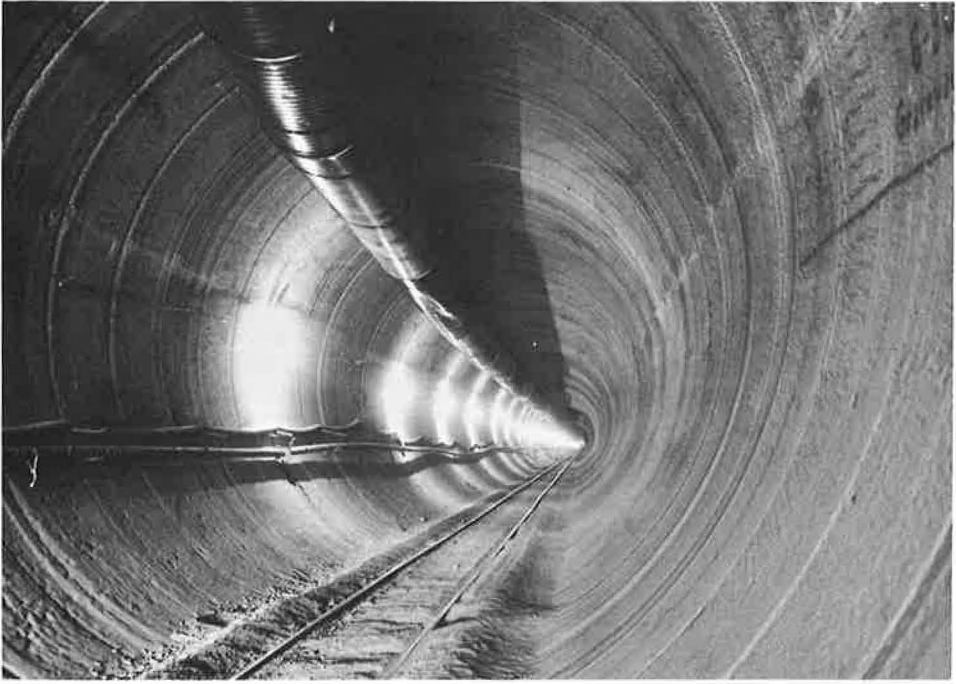
Figure 3. Tunnel 1 showing typical unsupported section.
