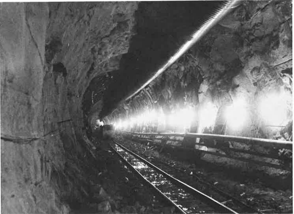
Figure 4. Tunnel 2 showing typical supported and unsupported sections.
