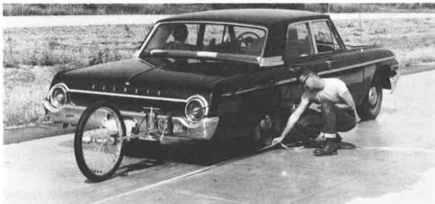
Figure 4. Measurement of observed stopping distance.
