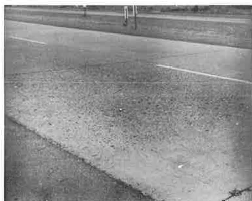
Figure 2. Concrete pavement surface deterioration.
