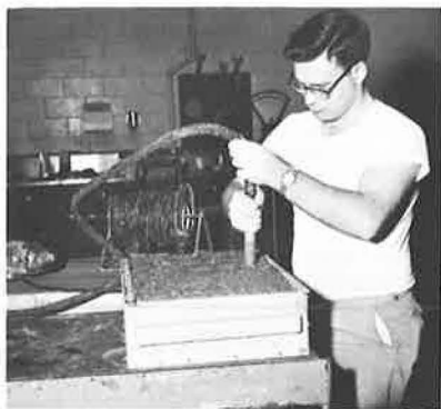
Figure 3. Vibration of test block.
