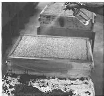
Figure 5. Fog spray being applied to concrete during delayed finishing process.
