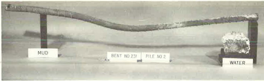
Figure 7. Condition of 1.10 x 1.37-in. oval reinforcing steel. Notations of "mud" and "water" are where the pile was in contact with those environments.
