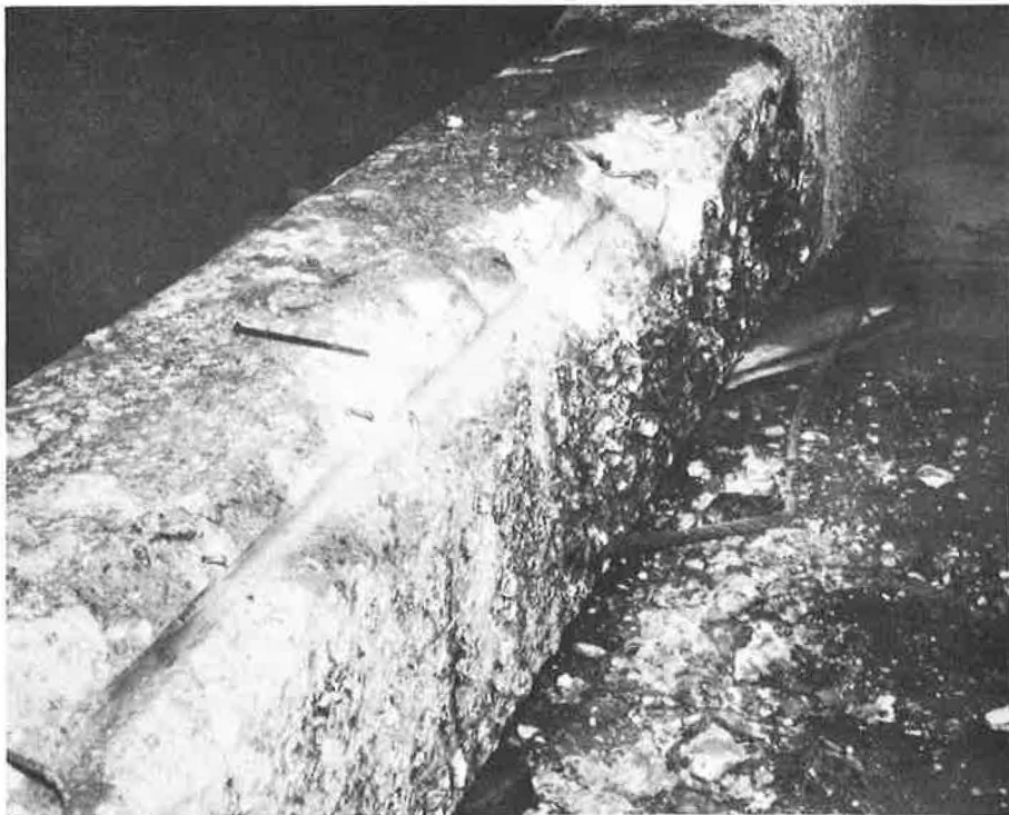
Figure 6. Corner of pile after removal of reinforcing steel.
