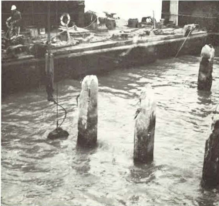
Figure 3. Excavating mud from base of piers—superstructure removed.
